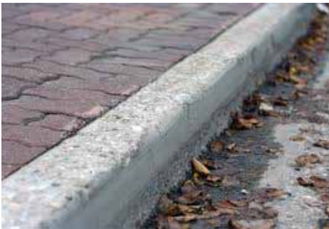
Concrete Curb and Gutter Concrete Paving
