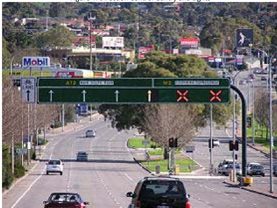
Figure 4: Direction Control Gantry and Lights
