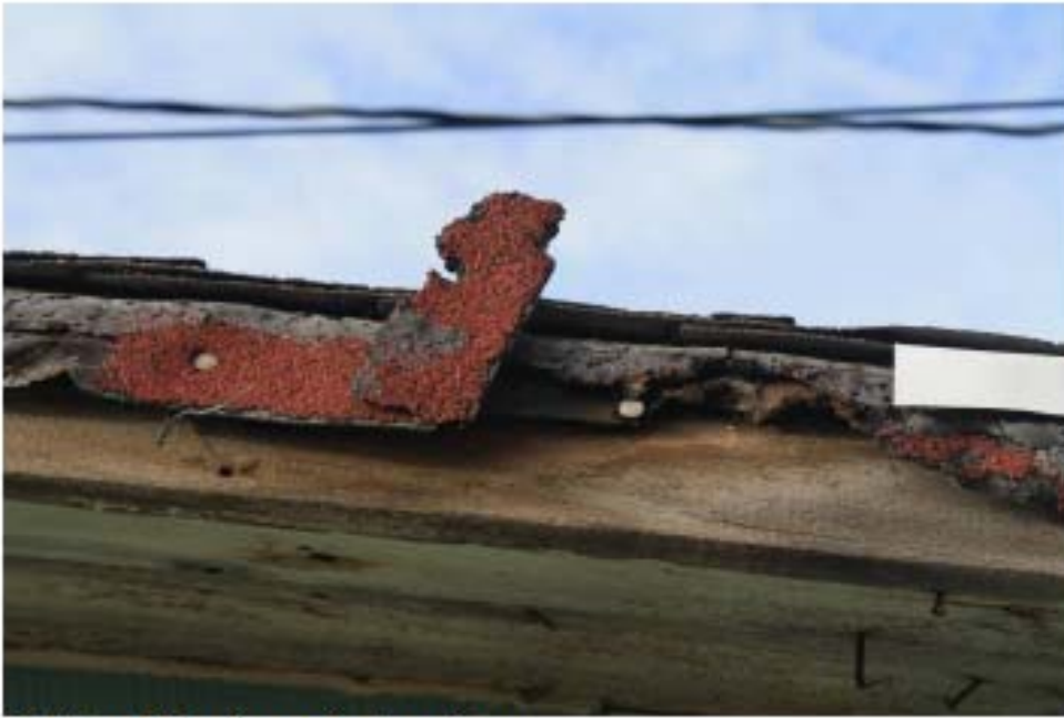
Soffit and fascia south elevation
