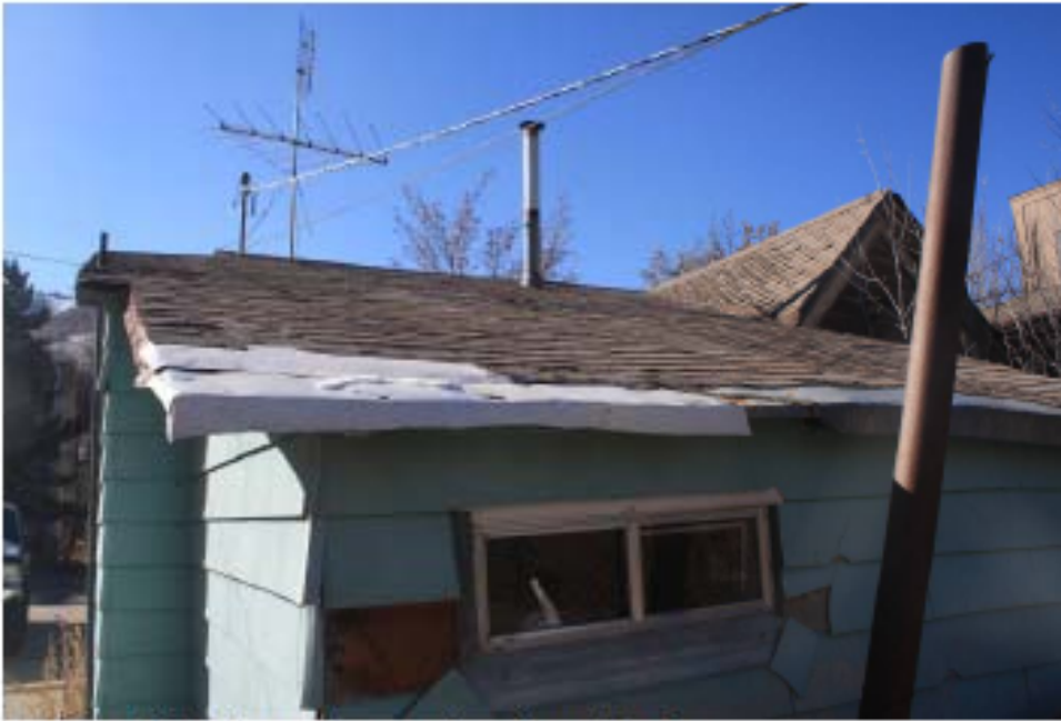
Soffit and fascia east- rear elevation. Roof penetrations.
