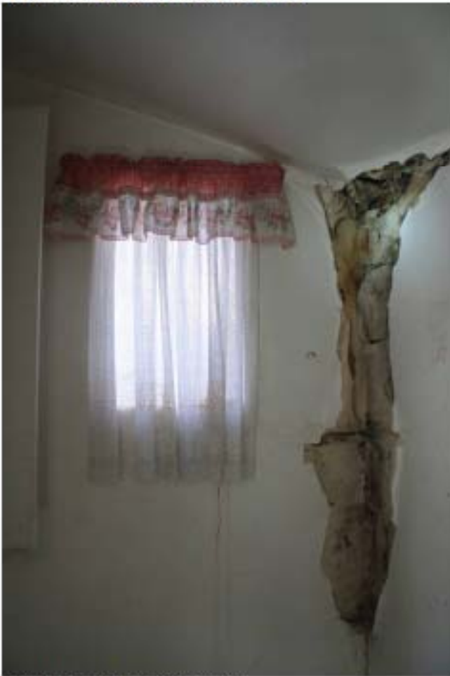
Interior northwest window
