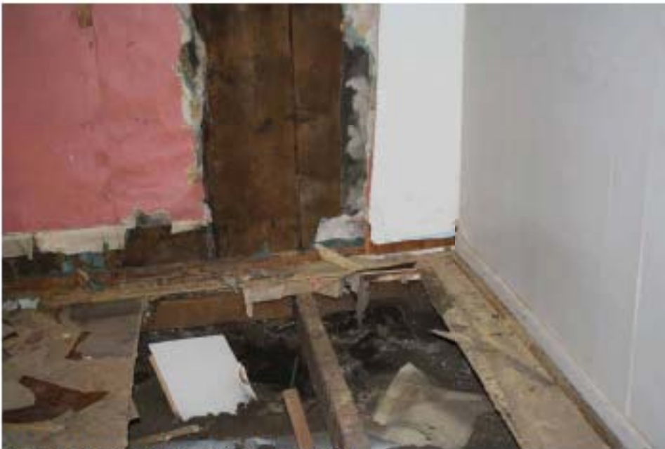
1.Look at interior excavation north wall
