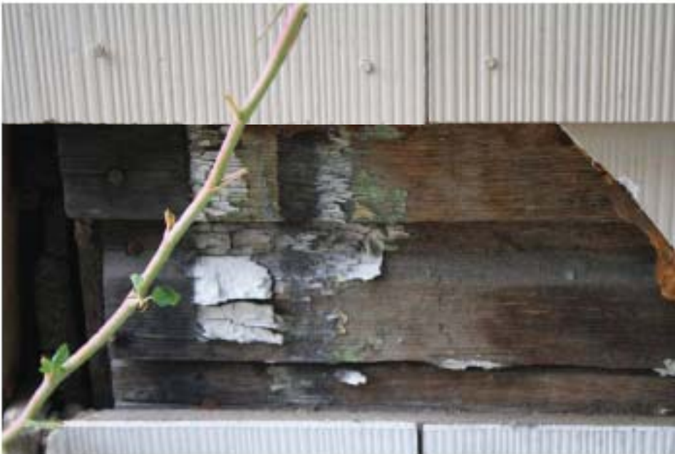
2. Siding detail northwest corner
