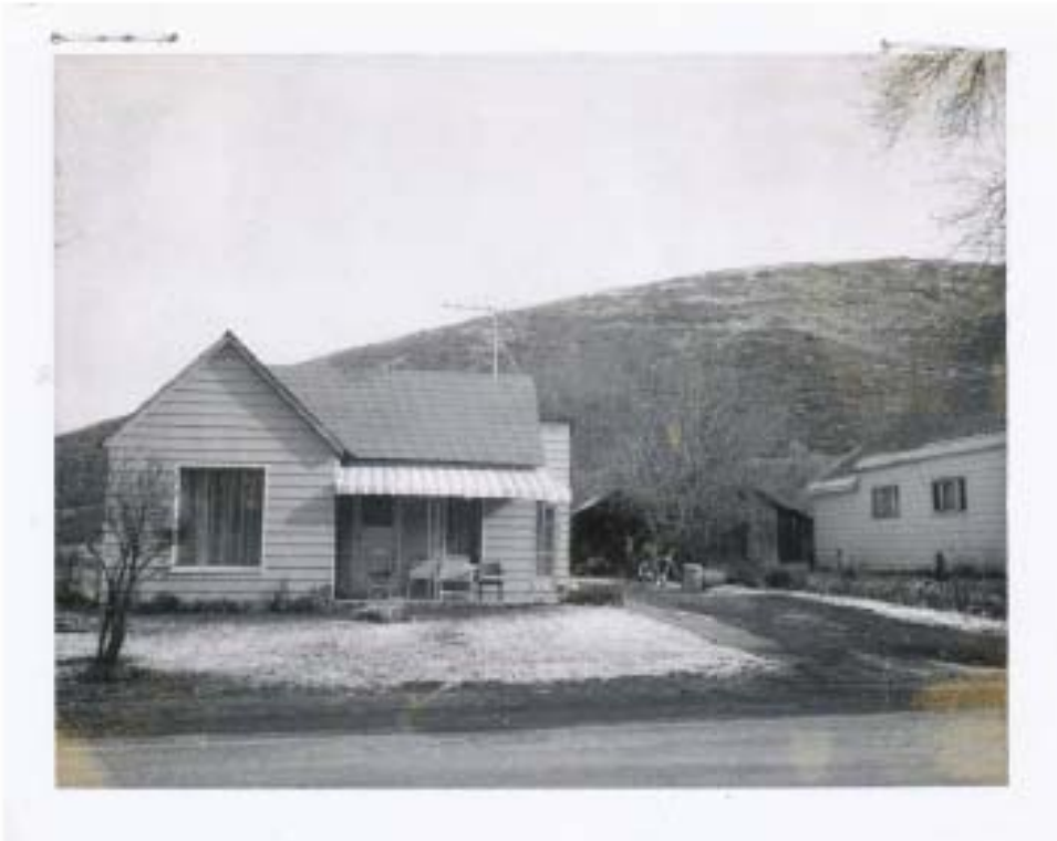
1958 photograph shows immature tree in front and driveway is not finished.
