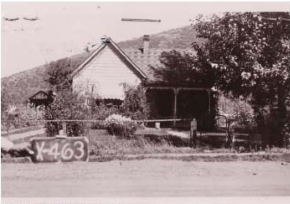
1450 Park Ave. Historic porch
