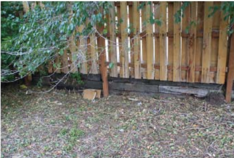
1.Railroad tie retaining wall
