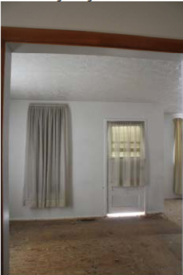
Ceiling lowered throughout house
