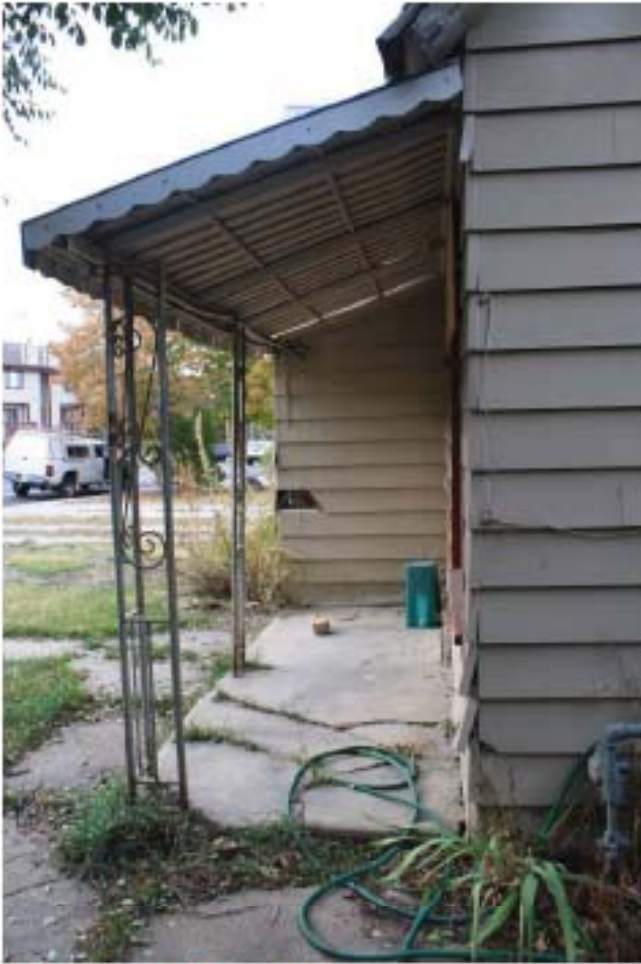
3. Porch- south elevation
