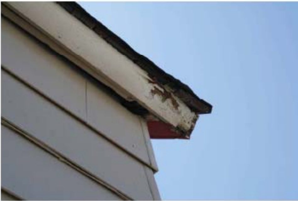
6.Fascia detail northeast corner
