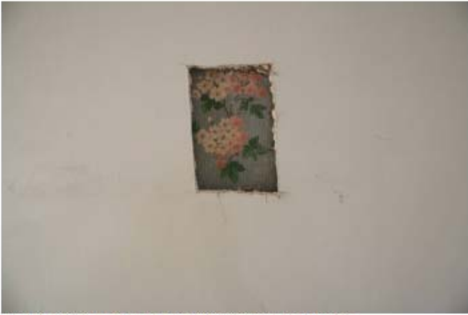
Wall structure- wallpaper on 1X12 vertical plank typical
