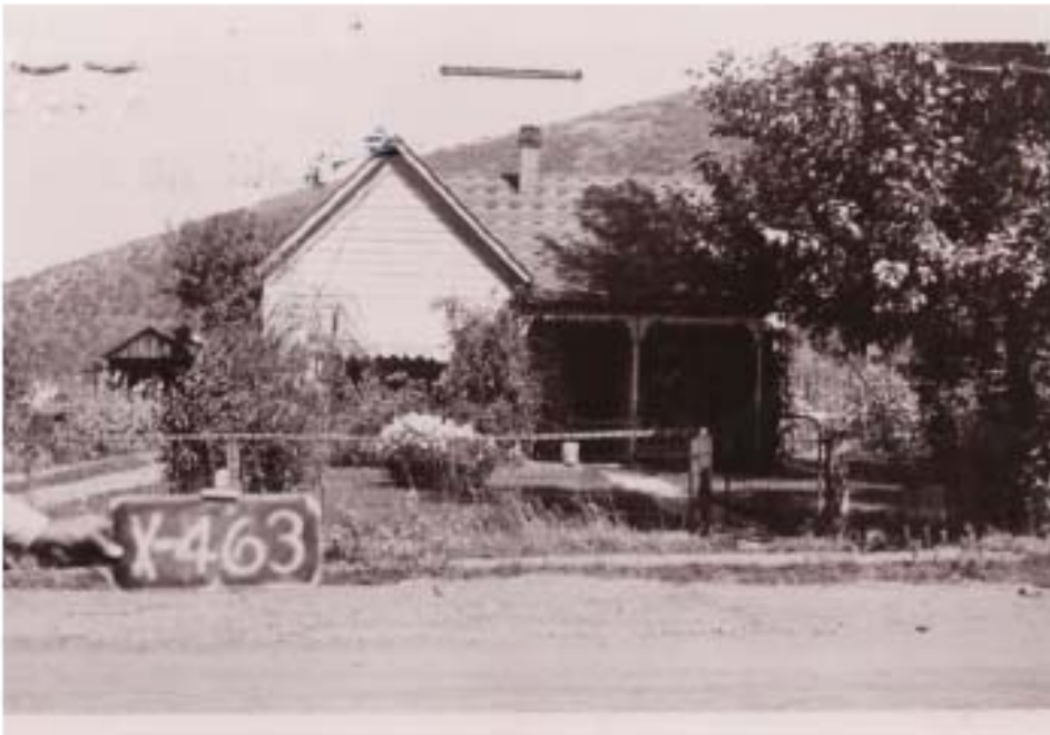
Historic front porch structure on 1450 Park Ave.
