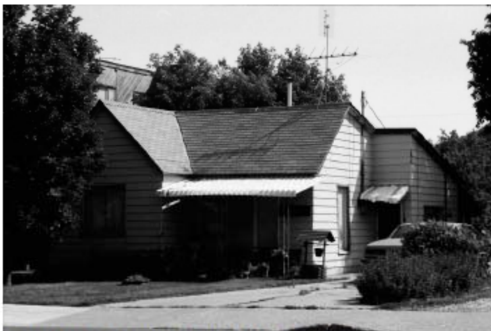
Older photo showing vegetation and concrete areas
