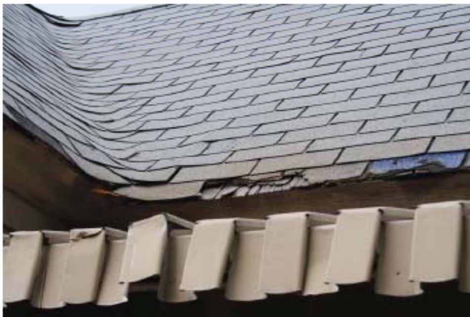
1.Original wood shingle
