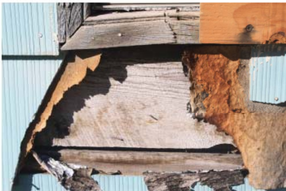
Typical 2" wood casing
