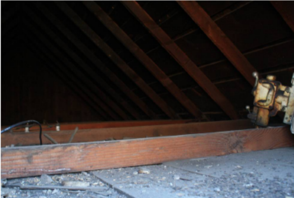
Roof and ceiling framing
