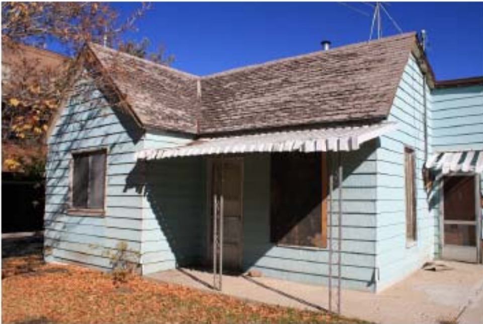
West primary façade- 2010 photograph
