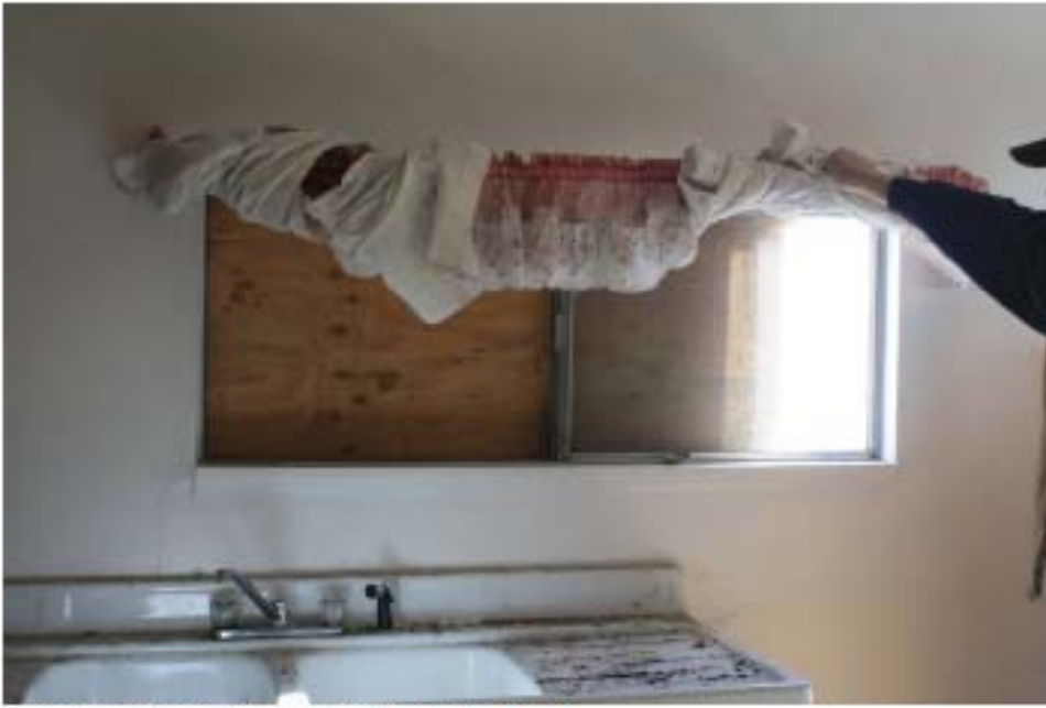
Interior kitchen window casing modified
