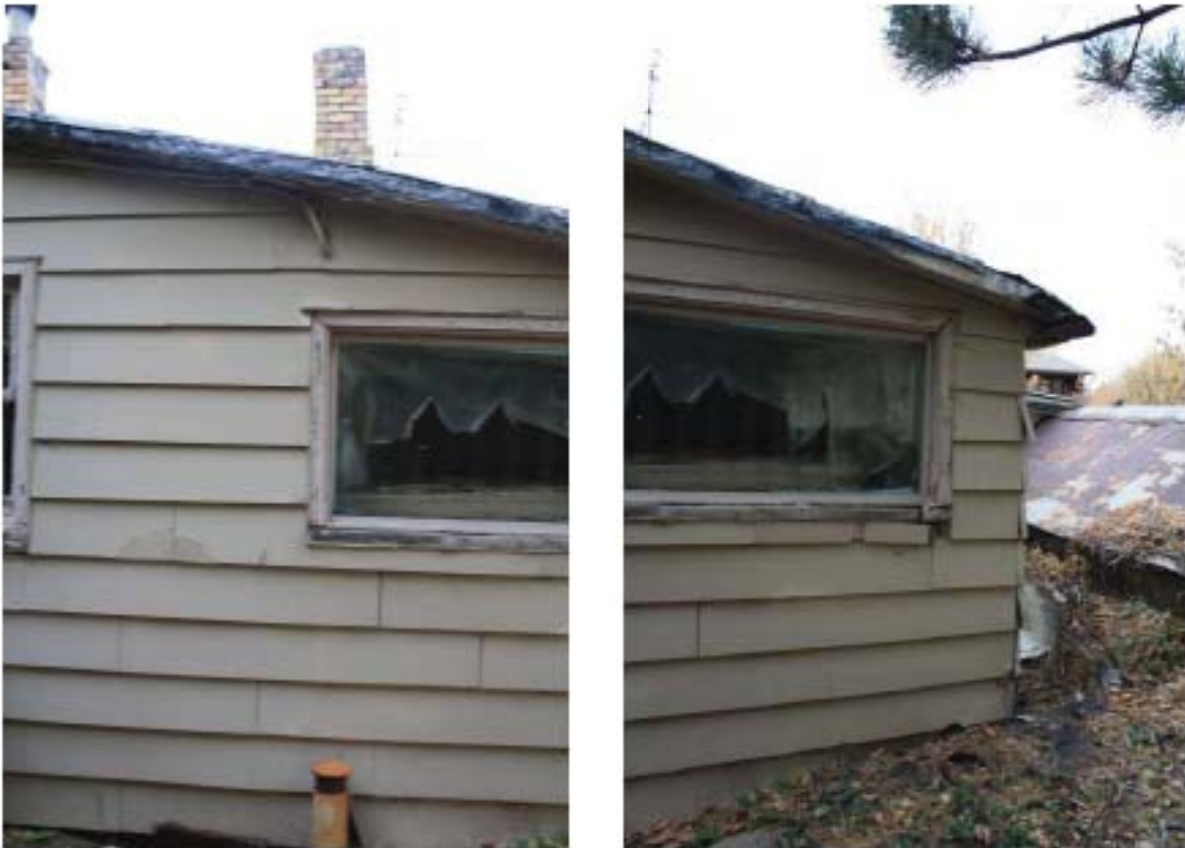
There is a large fixed single pane window in the mechanical room. It is 3'-3" off the ground and 4'-8" W X 2'-2" H. It has similar jamb and sill detail shown above.
