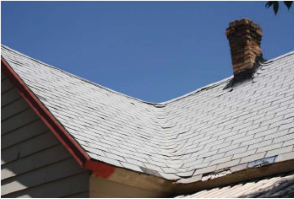
4.Original roof valley and chimney
