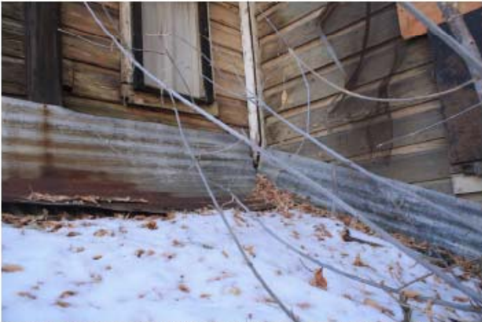
Mechanical shed roof- original siding material- north elevation
