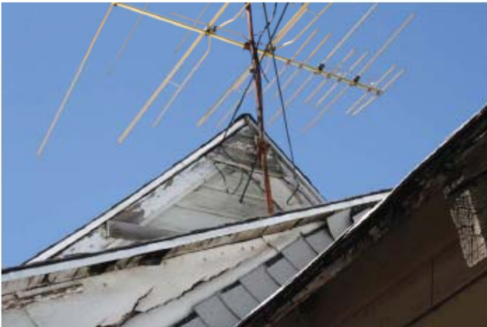
5.East elevation original gable
