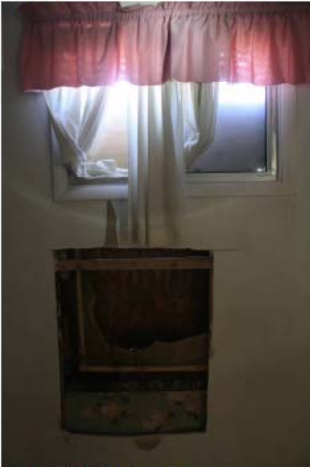
Interior east bedroom window
