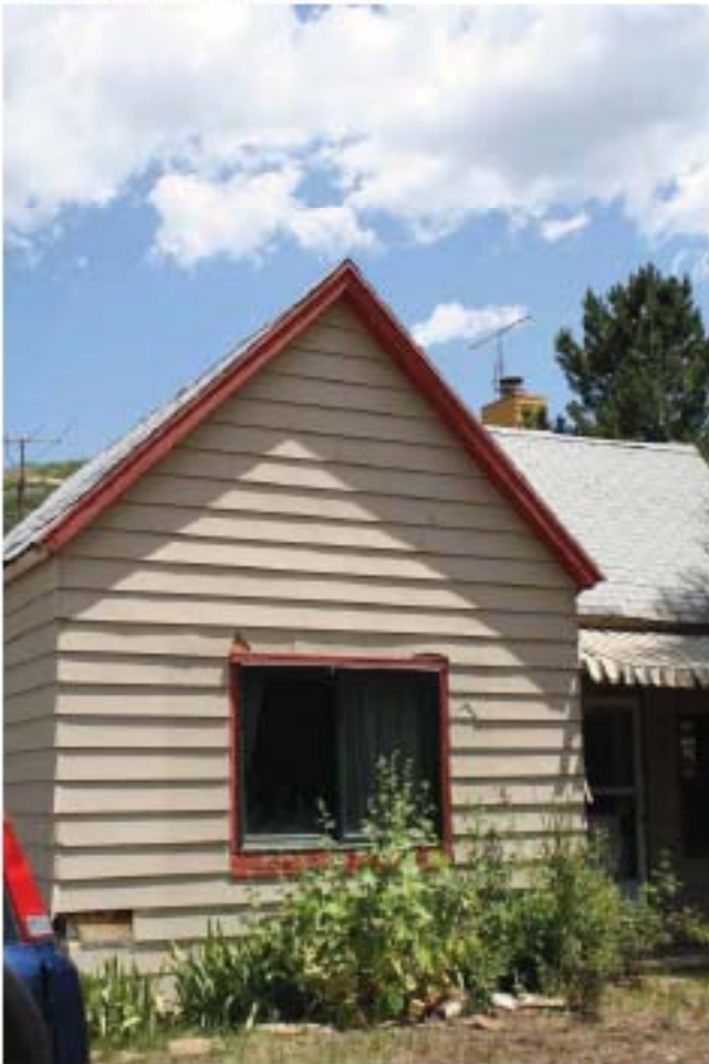
3.Original west gable
