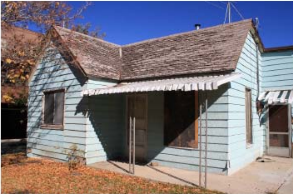
West front porch-2010
