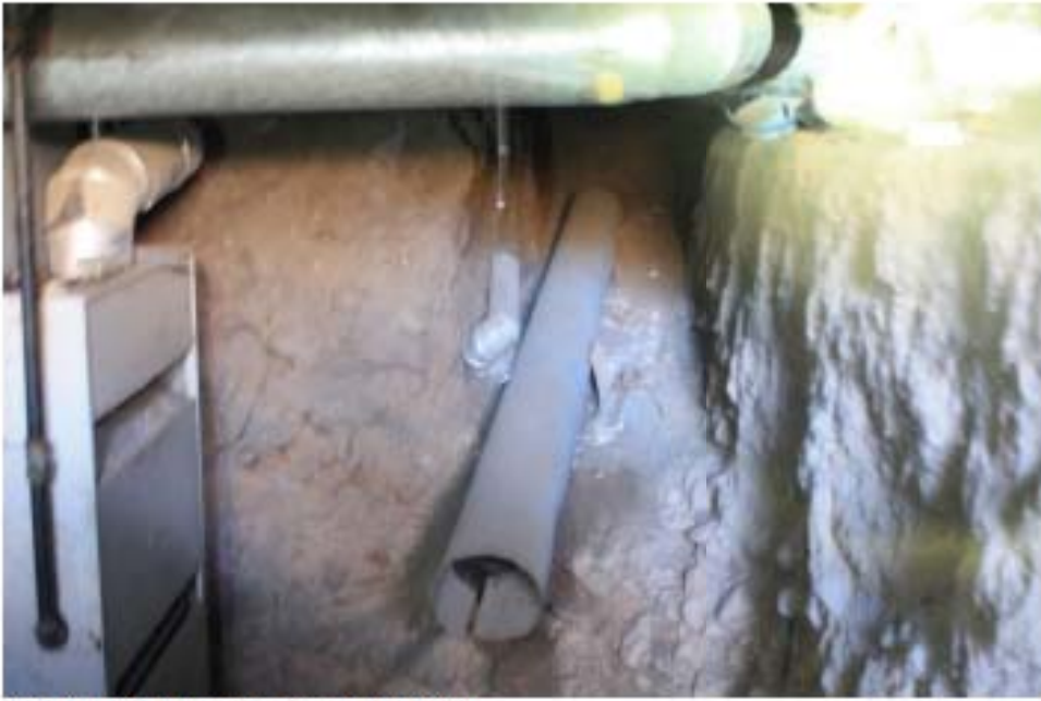
Duct work through excavated dirt
