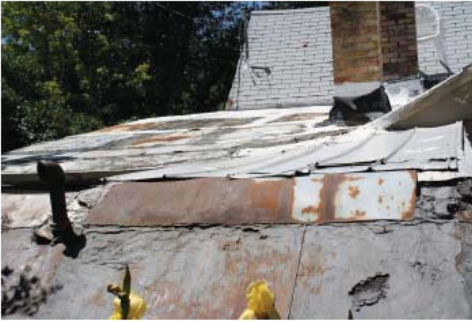
8. East elevation roof condition and chimneys
