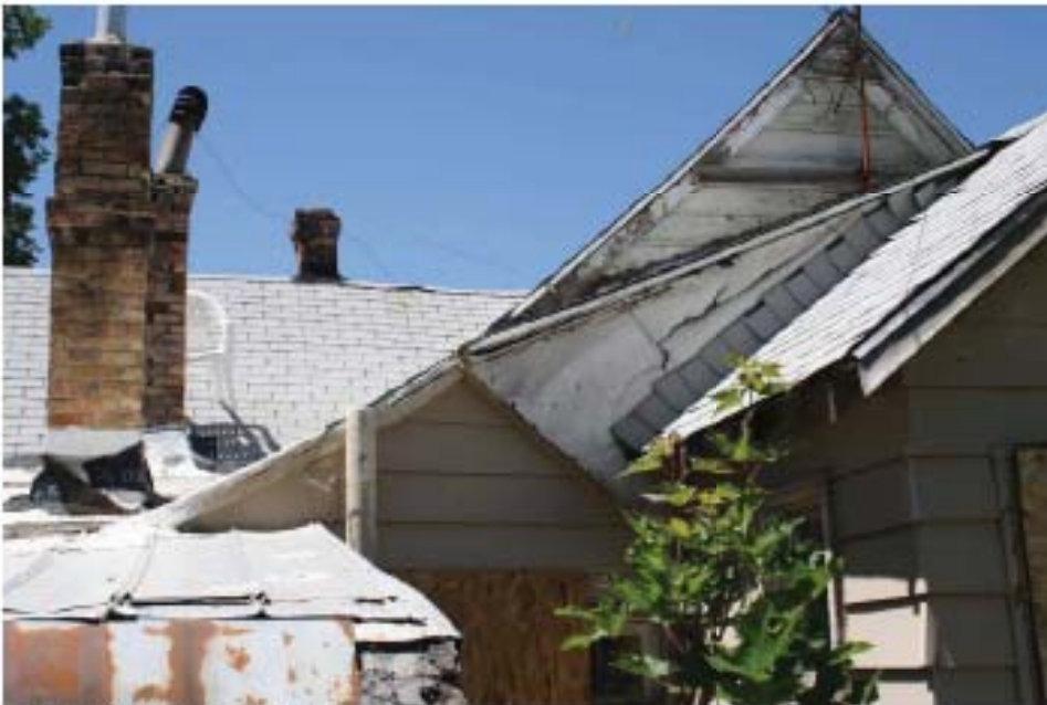
7. Toilet plumbing vent.
