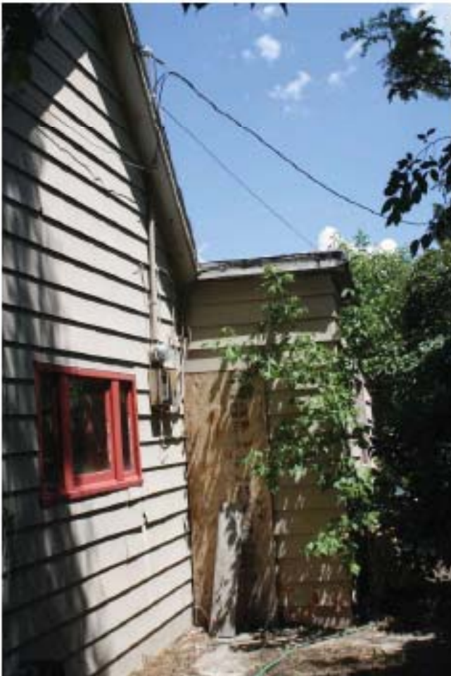
5. West kitchen door
