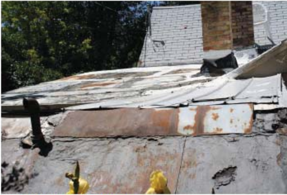
Root cellar roof in foreground.
