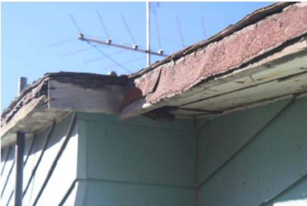
Soffit and fascia southeast corner kitchen/bathroom
