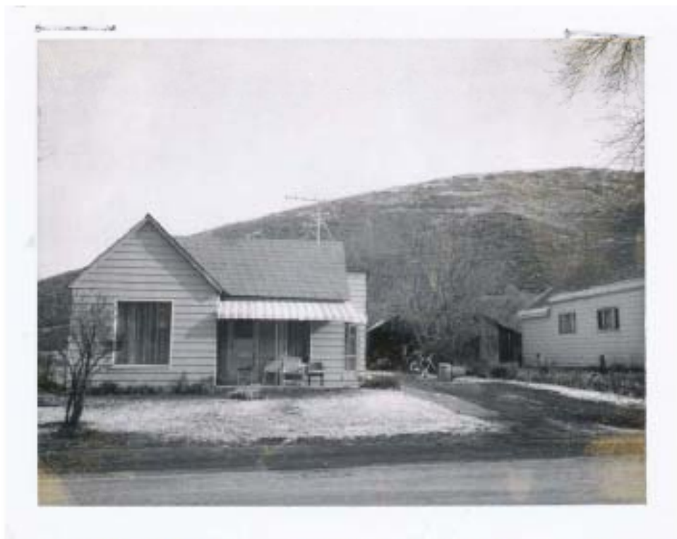
1958 Photograph-shows many of the modifications made to the historic house West primary façade
