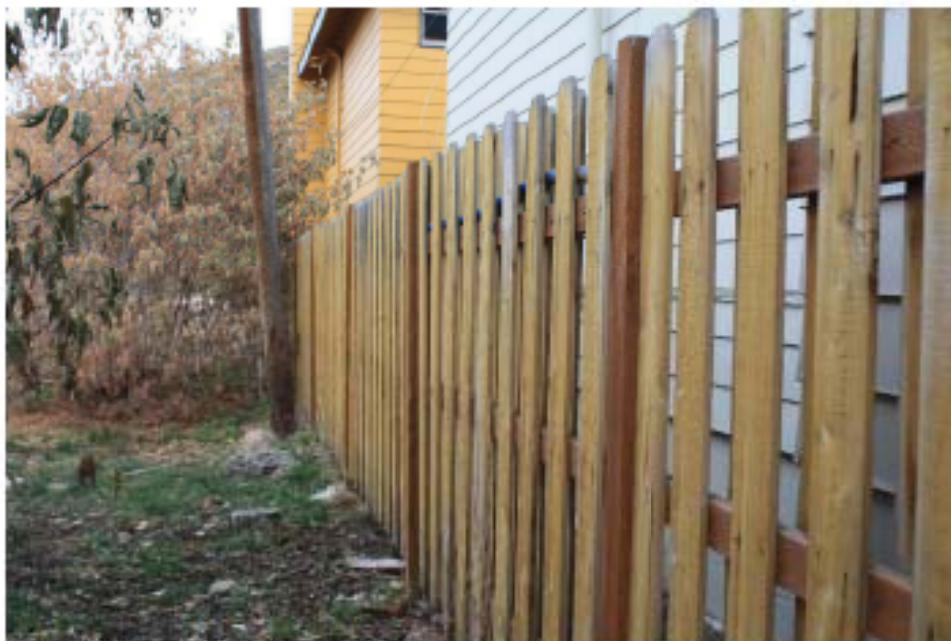
1.South property line wood fence
