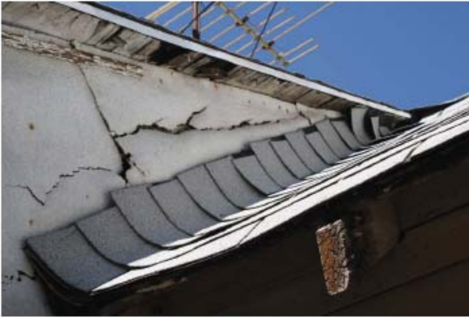
6. East elevation overbuild at bathroom
