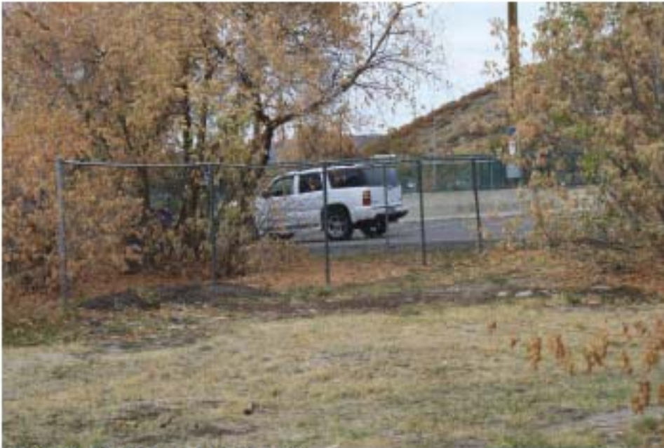
2. Chain link fence rear northeast
