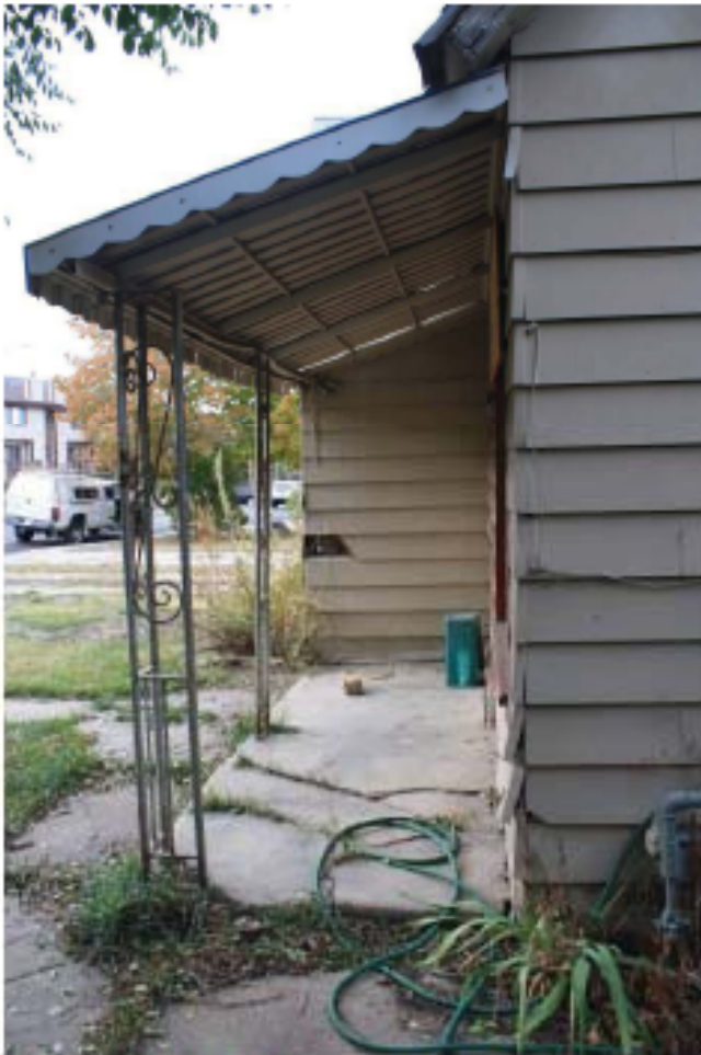
1.Original porch intersection-southwest corner
