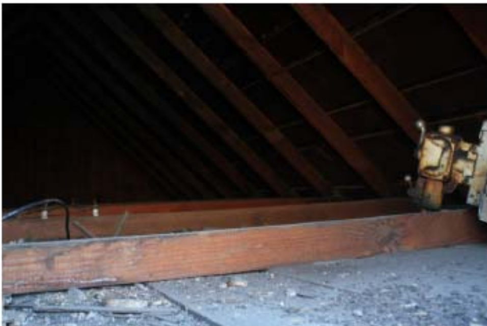
Knob and tube cloth wire-typical
