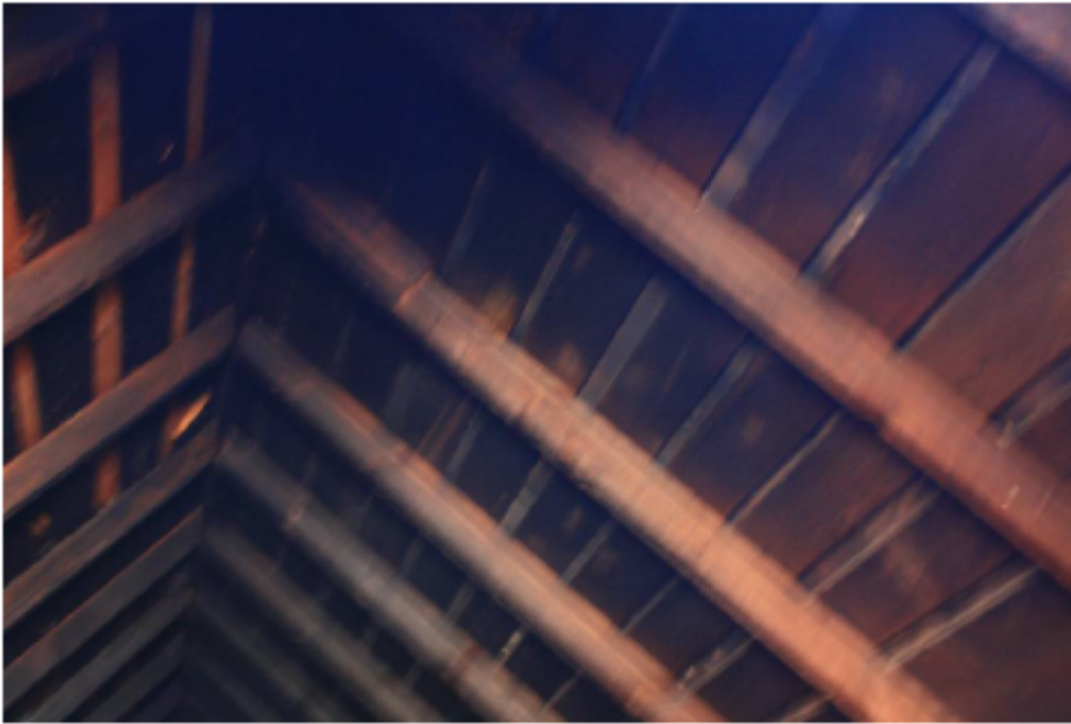
East-west gable framing
