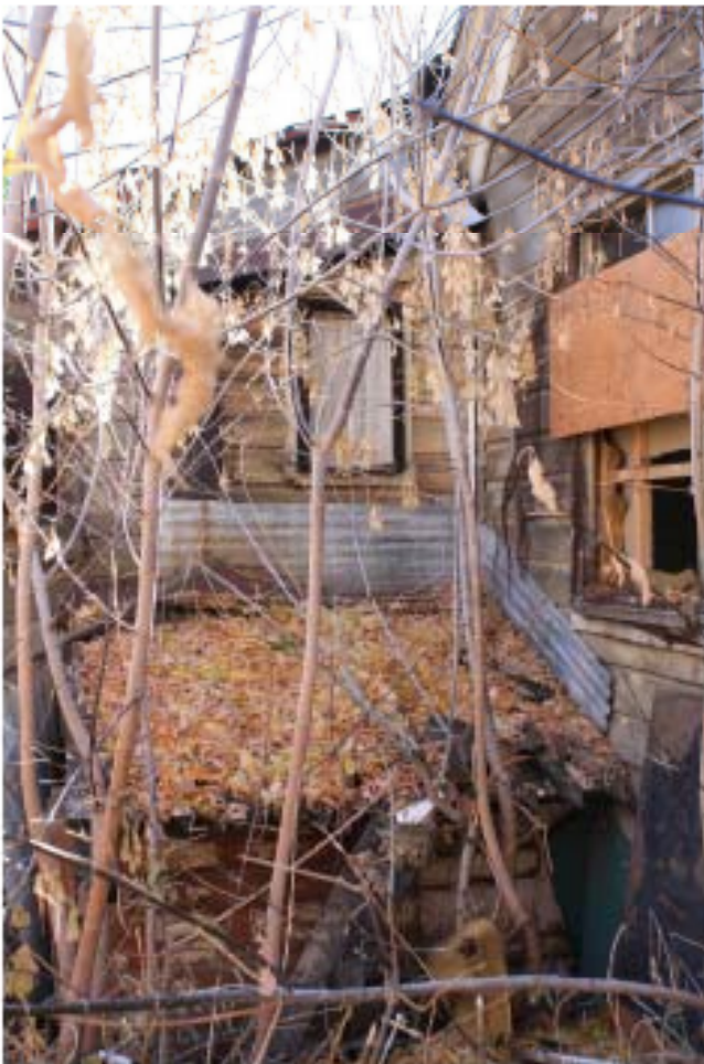
North elevation-shed access to mechanical
