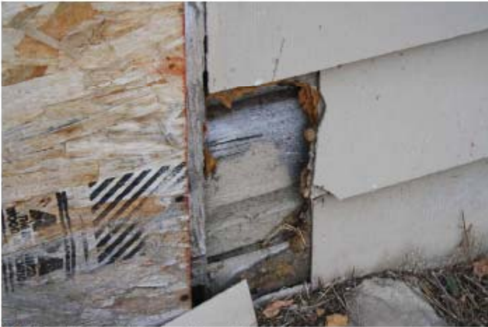
6. Siding detail-northwest gable north elevation
