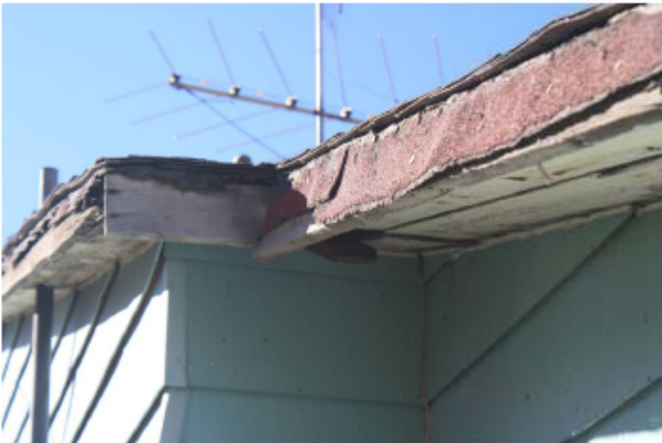
Transition from 6" overhang to 10" overhang
