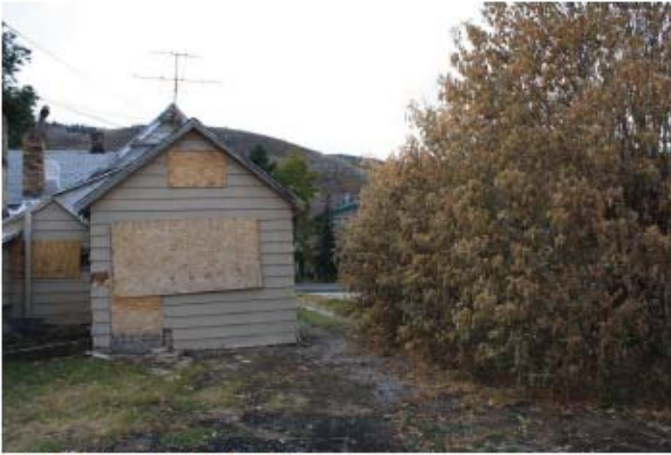
5. Northeast gable-north façade
