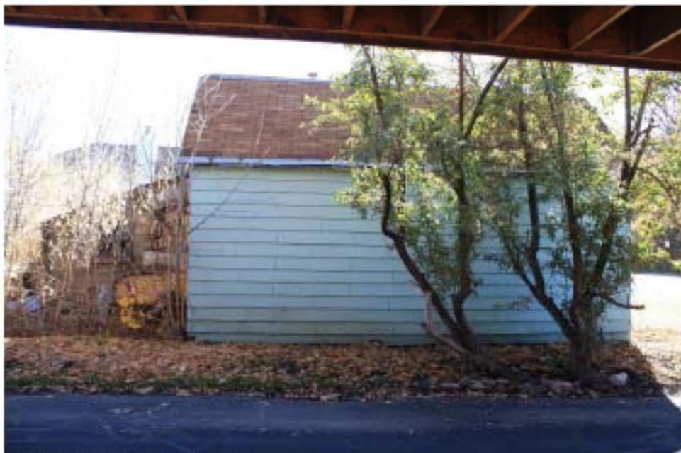
East-west gable roof
