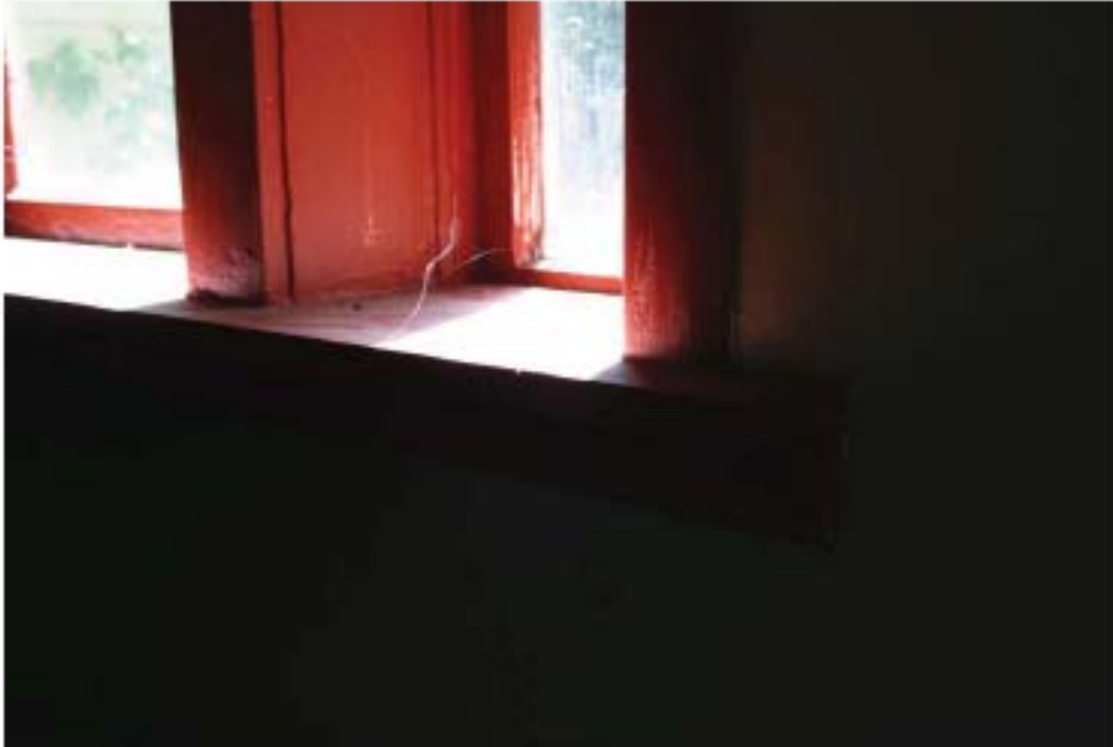
Interior of window detail.
