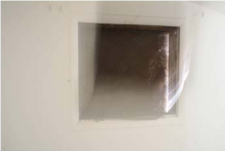
Northeast window-modified frame
