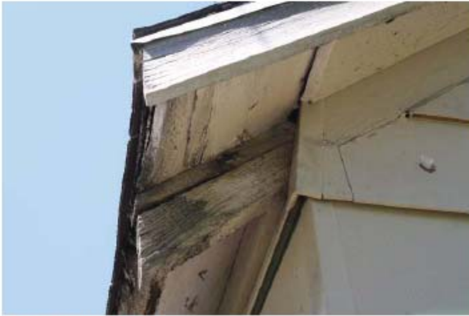
2.Soffit detail northwest corner
