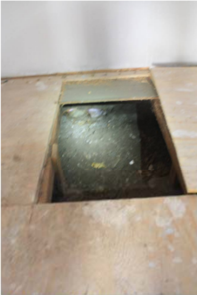
Dirt and rubble foundation-typical
