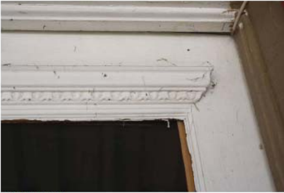
Front door detail.
