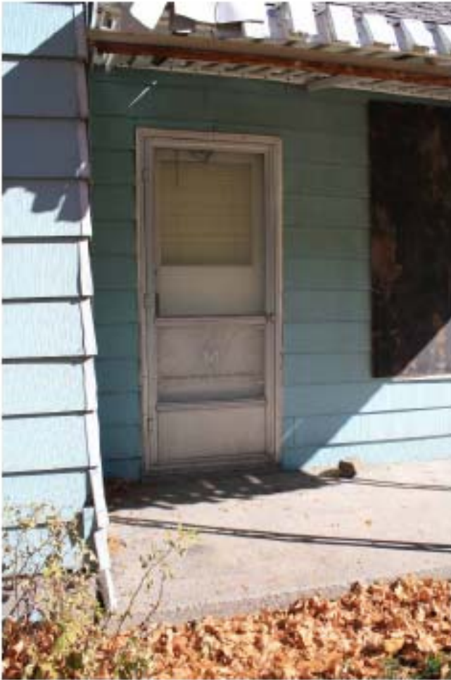
Concrete slab porch floor
