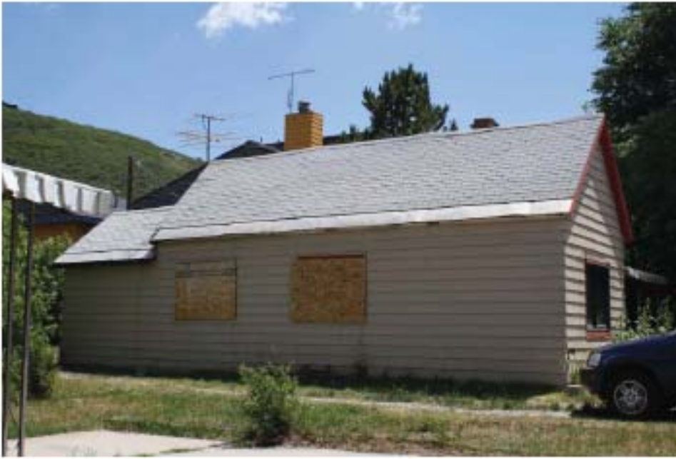
1. North elevation (chimney and roof of project to the south seen)
