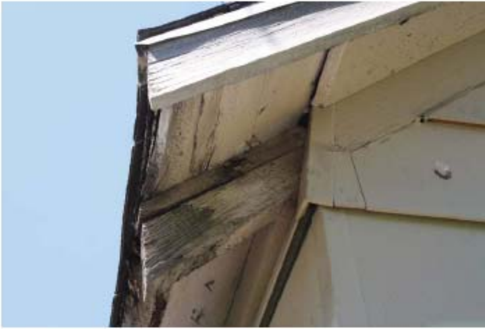
5.Soffit and fascia northwest corner
