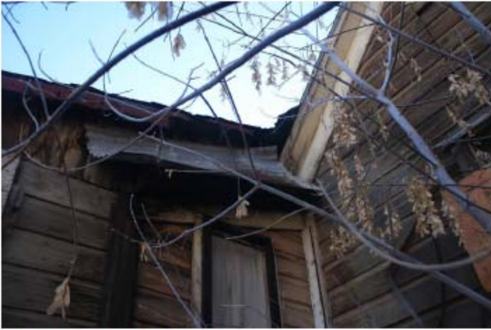
Corner- original 4'-0" shed structure
