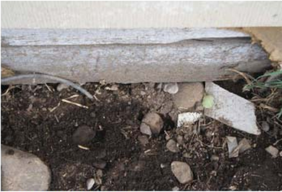
1.Foundation rubble-north elevation
