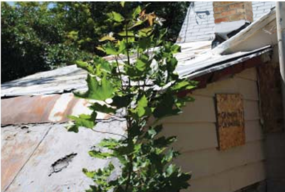
Window at stair to root cellar.
