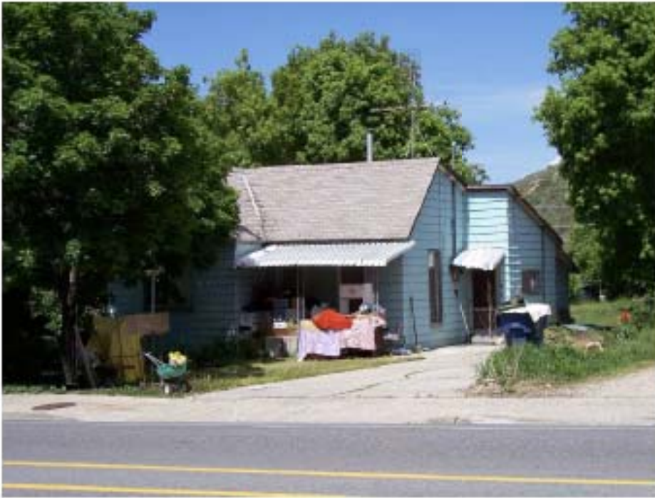
West primary façade 2006 photograph
