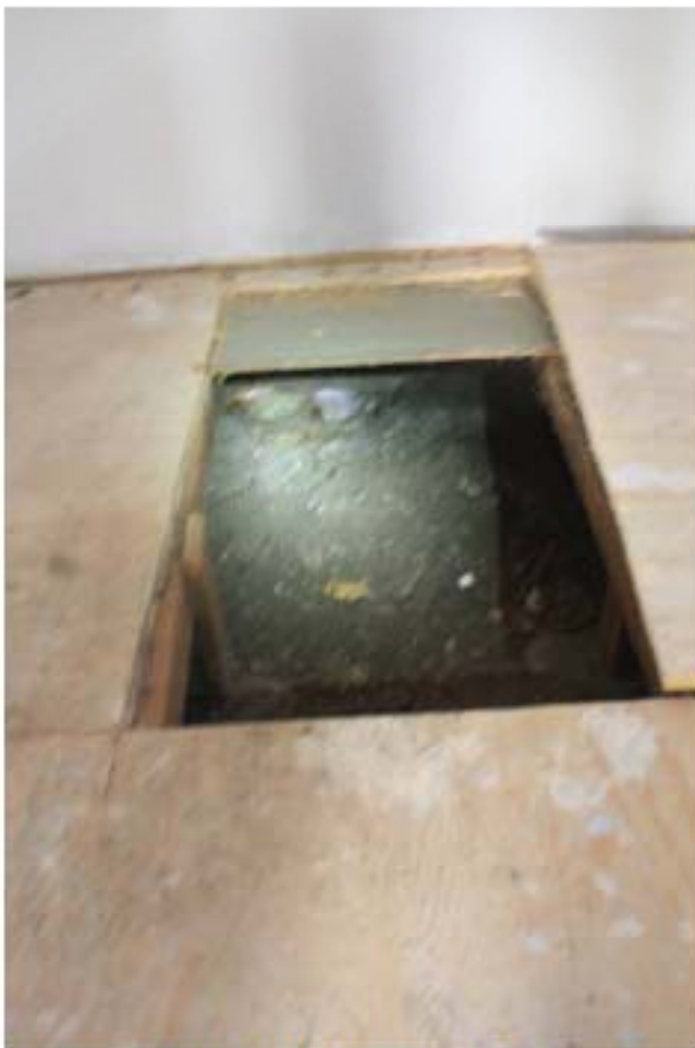
Foundation-floor joist on rubble stone
