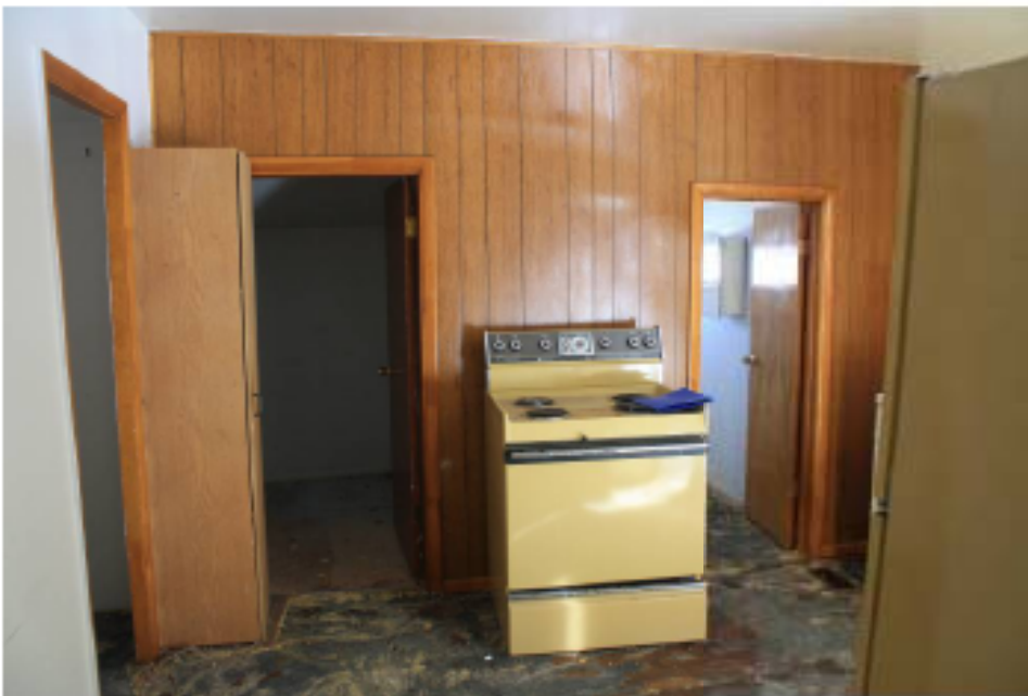
Typical interior door and casing
