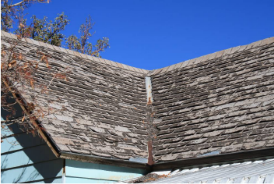
Intersection-valley east-west gable and north-south gable
