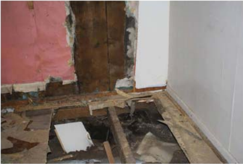
1. 1X12 wall construction. 2 1/8"X6" floor joist.
