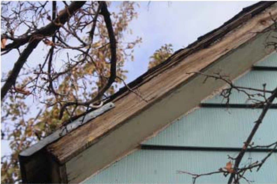
Typical soffit and fascia-functional and simple
