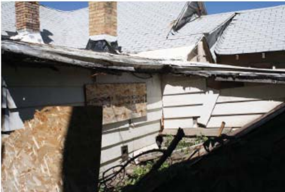
2. East elevation mechanical room shed
