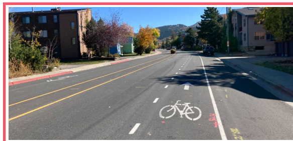
Park Ave Bike Lane & Shared Street | Deficient
