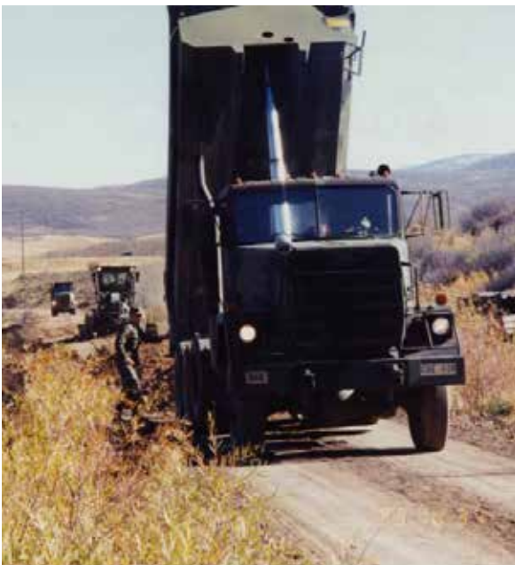
Construction of the Rail Trail
