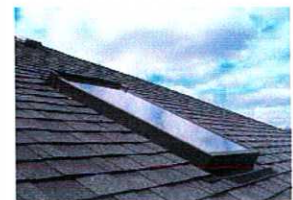
Skylight placed flush to roof
