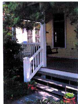
Appropriate porch detailing
