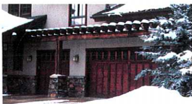
Not this - Garage doors for three cars occur on the same wall plane
