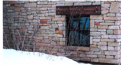
Window is a feature element within this wall plane
