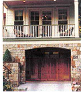
Patio over garage lessens its visual impact
