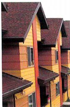
Roof overhangs protect walls
