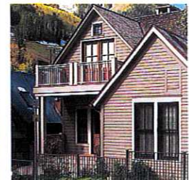
Porch roof breaks up two story element
