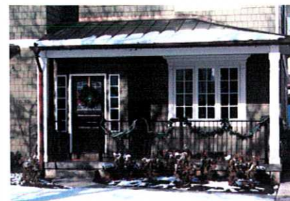
Porches are elevated 18” above finished grade
