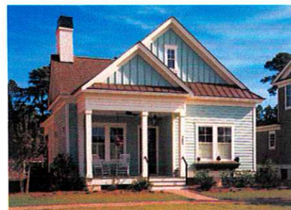
Porch roof forms are consistent with home
