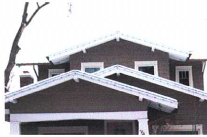
Appropriate roof overhangs
