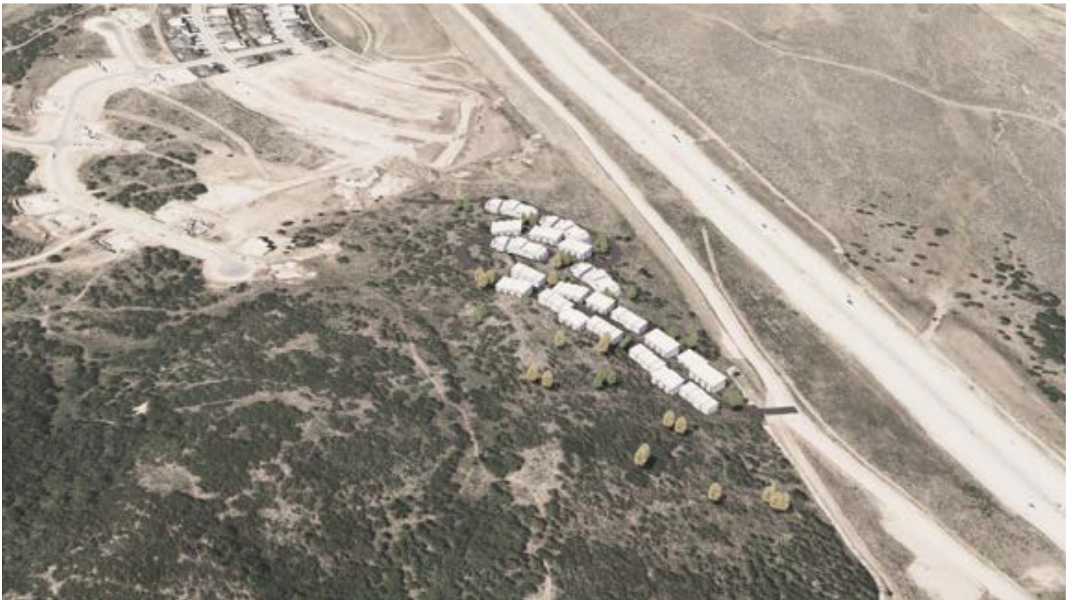
illust. 44.2 - south birdseye view looking north east towards the junction of hwy 248 & hwy 40 (Stereotomic )
