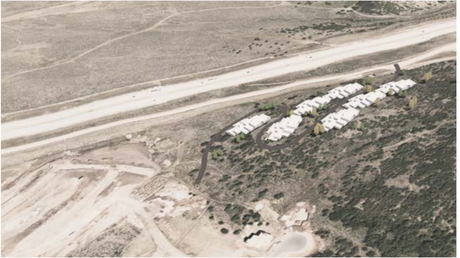
illust. 51.1 - West view of the massing as it relates to the lower hillside (Stereotomic )
