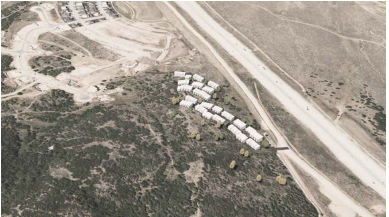
illust. 36.2 - south birdseye view looking north east towards the junction of hwy 248 & hwy 40 (Stereotomic )
