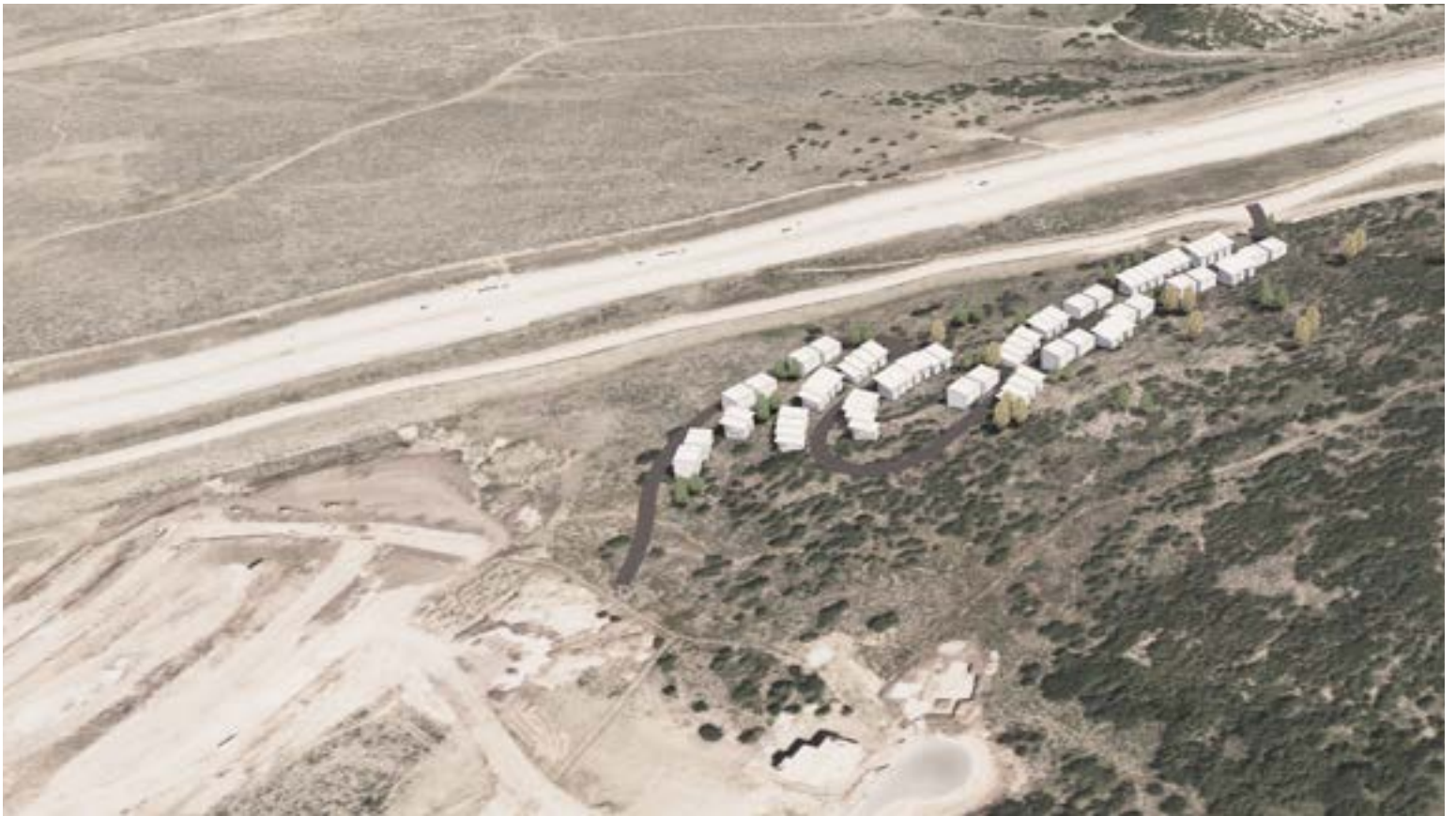
illust. 37.1 - West view of the massing as it relates to the lower hillside (Stereotomic )
