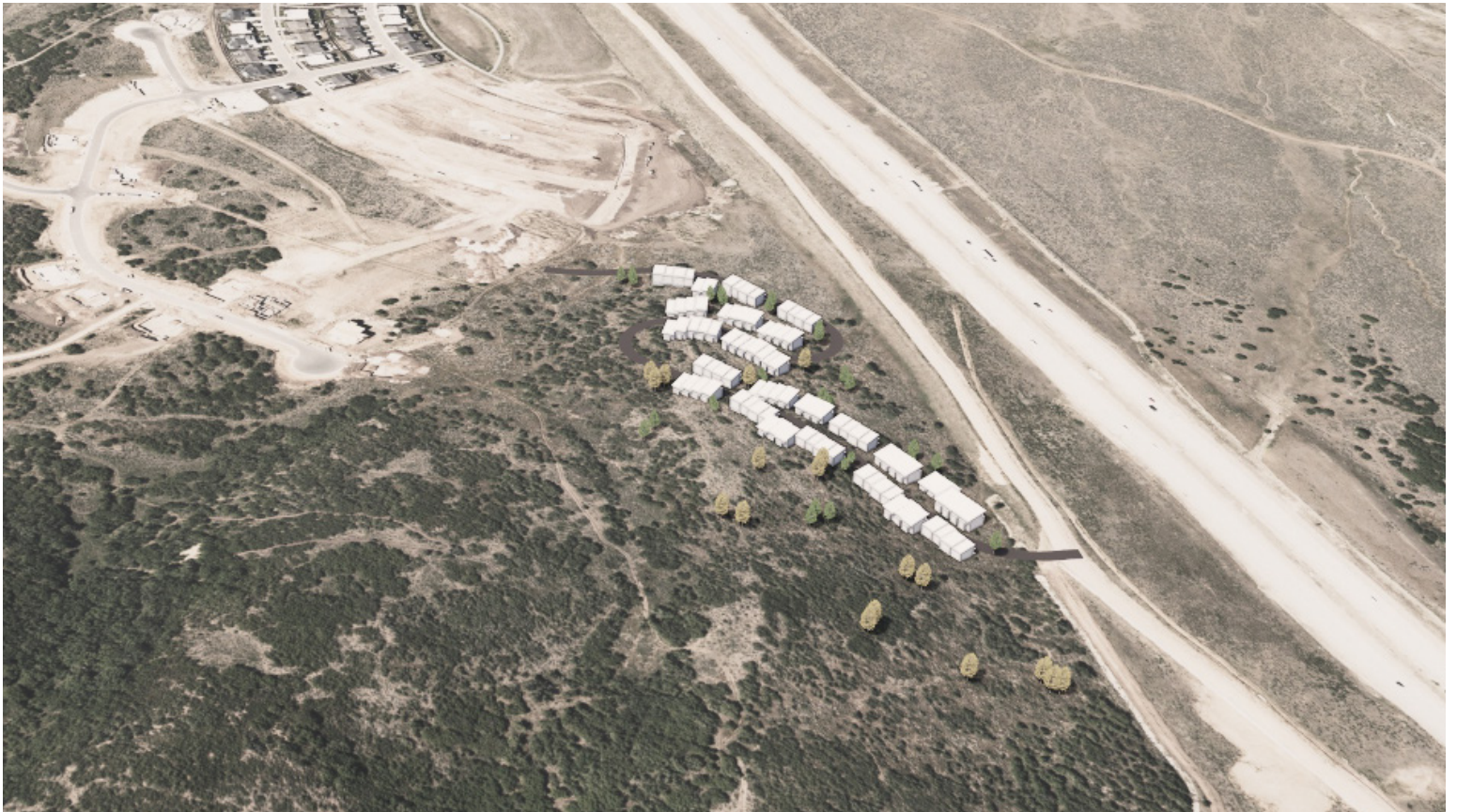
illust. 36.2 - south birdseye view looking north east towards the junction of hwy 248 & hwy 40 (Stereotomic )
