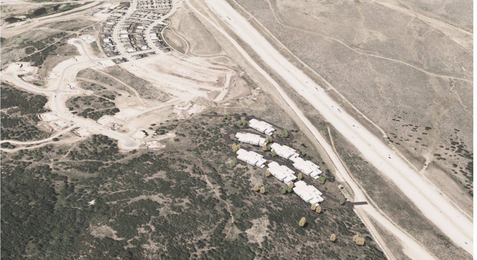
illustr. 50.2 - south birdseye view looking north east towards the junction of hwy 248 & hwy 40 (Stereotomic )
