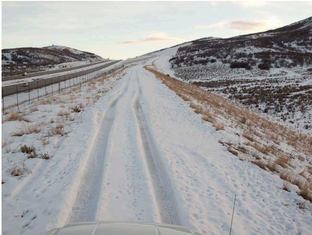
Photograph 11. US 40 and right-of-way fence, looking south along a frontage road from the east side of developable property.
