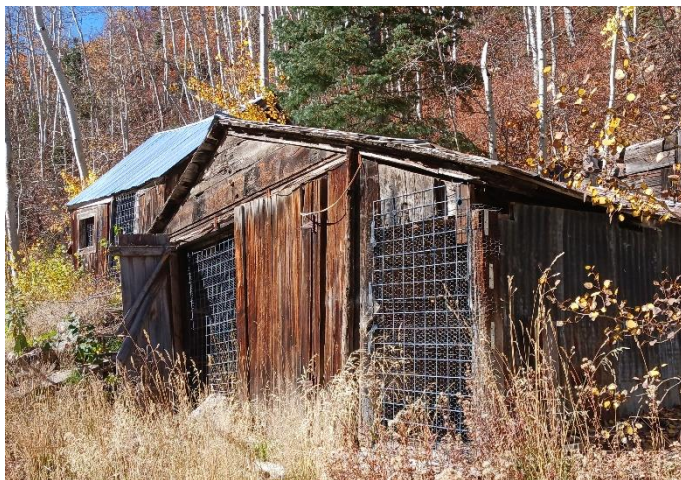
Figure 4: October 18, 2022 Photograph of Garage, front oblique.
