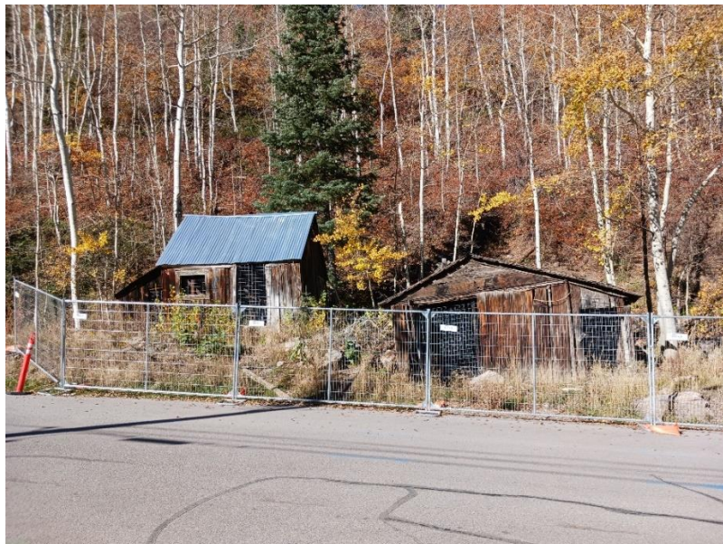
Figure 2: October 18, 2022 Photograph of Cabin and Garage, looking west across Daly Avenue.
