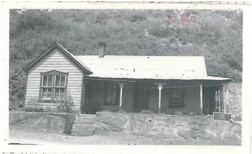
Figure 1: Tax card photograph of 1896 cross-wing cottage. Demolished 1984.
