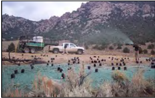
Seed can also be applied in a slurry with fertilizer and mulch to aid in native establishment while preventing erosion and weed growth.
