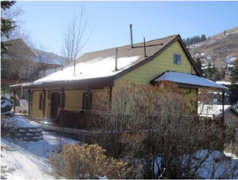
244 Sandridge Avenue. Northeast oblique. November 2013.
