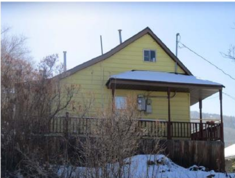
244 Sandridge Avenue. North elevation. November 2013.
