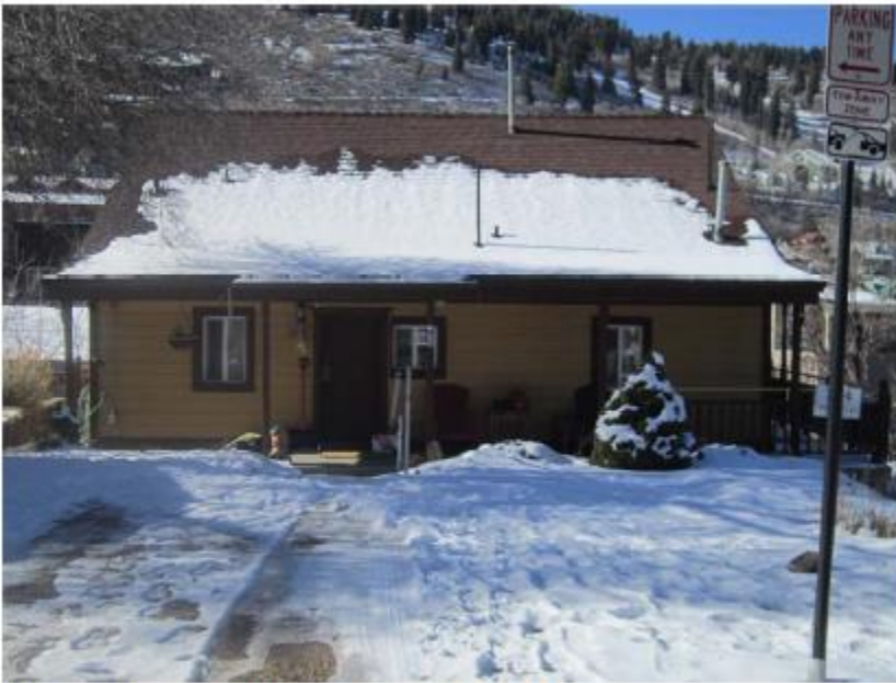
244 Sandridge Avenue. East elevation. November 2013.
