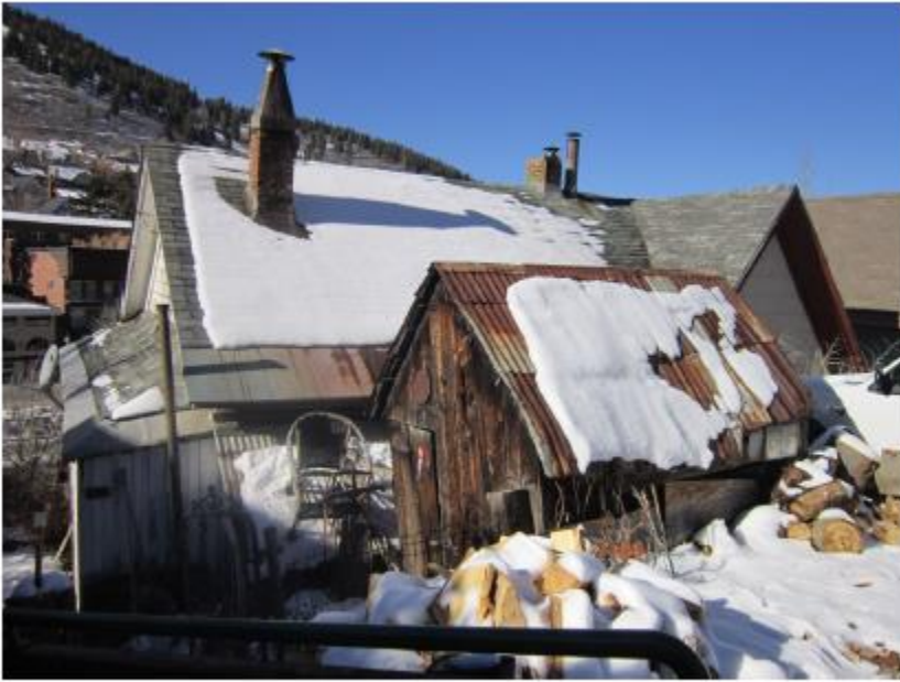
222 Sandridge Avenue. Southeast oblique. November 2013.
