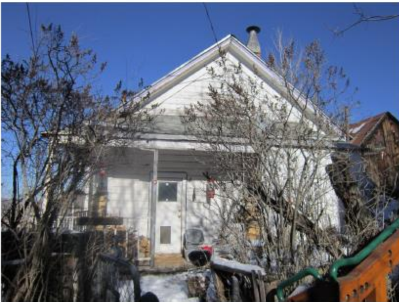
222 Sandridge Avenue. South elevation. November 2013.
