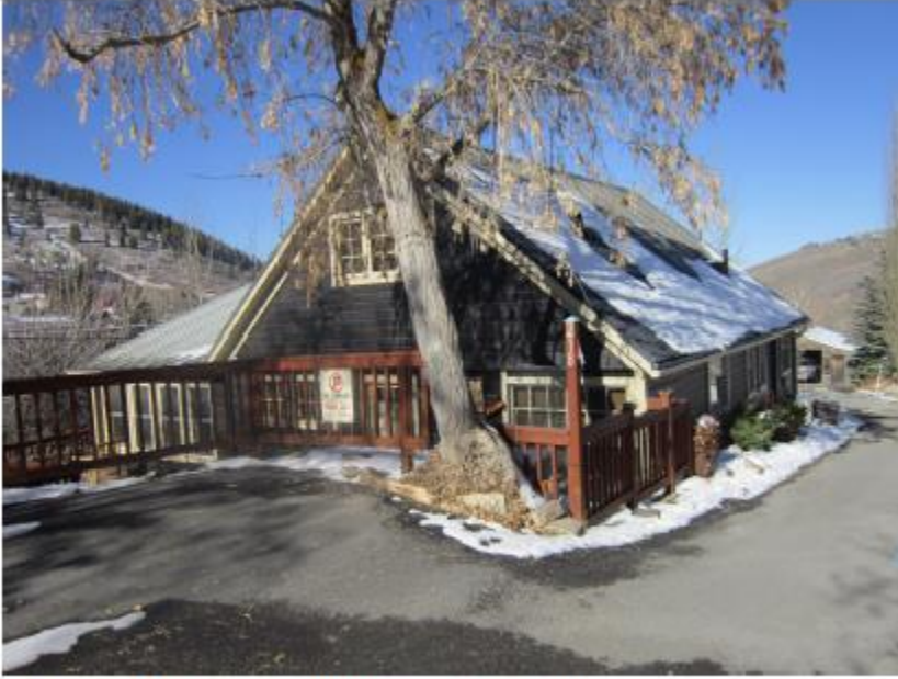
218 Sandridge Avenue. Southeast oblique. November 2013.
