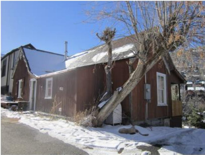
164 Sandridge Avenue. Northeast oblique. November 2013.
