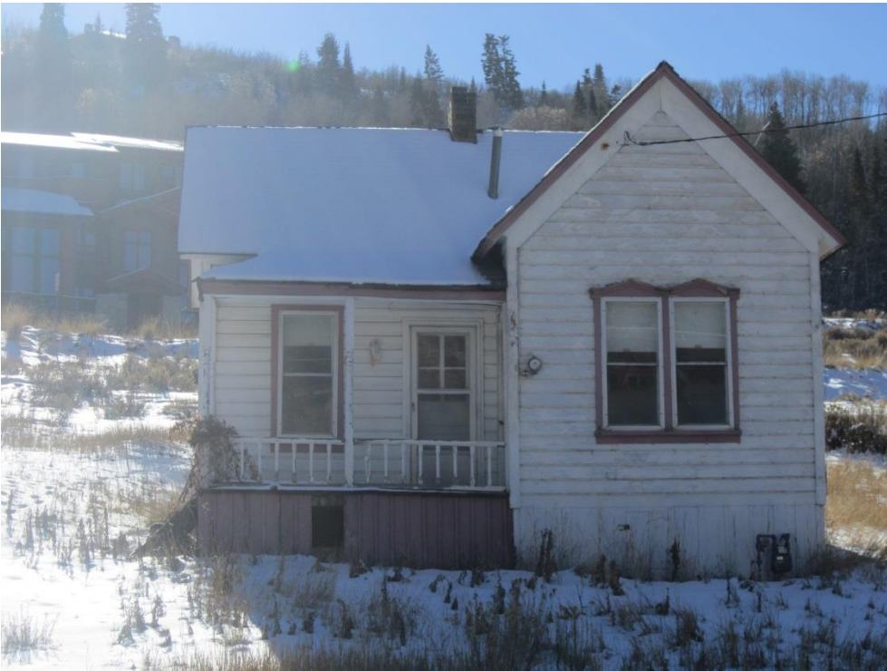
652 Rossie Hill Drive. North elevation. November 2013.
