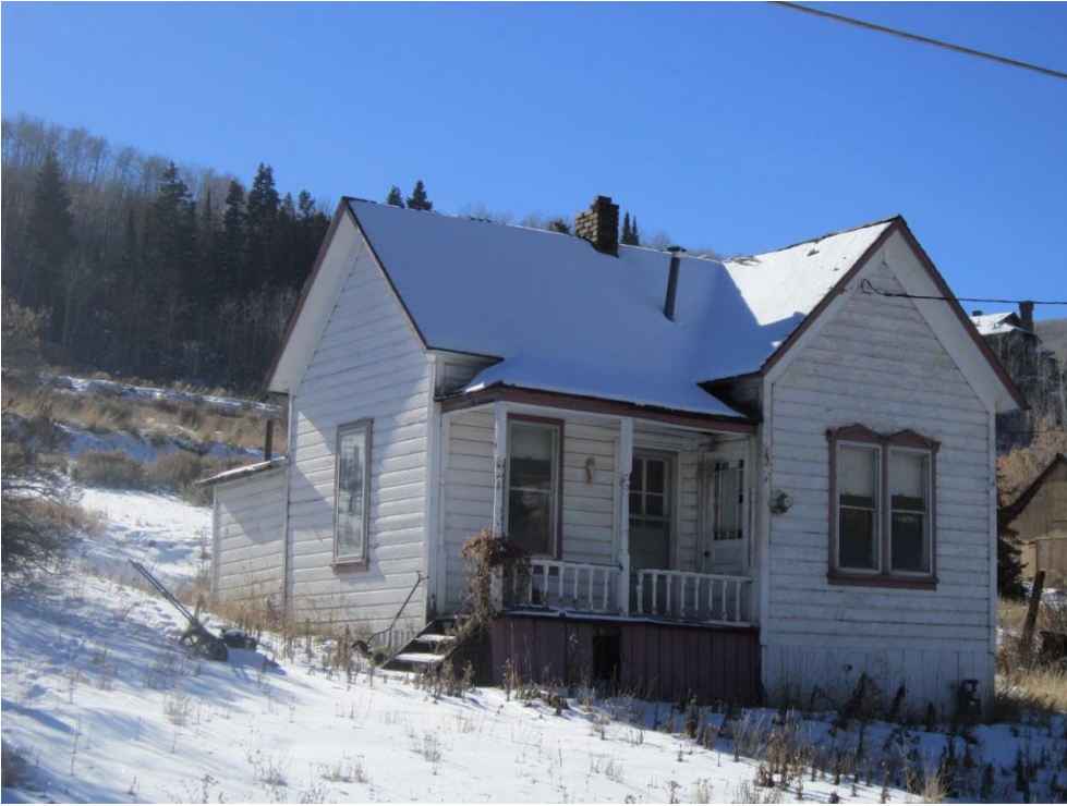
652 Rossie Hill Drive. Northeast oblique. November 2013.
