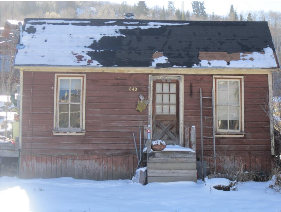
660 Rossie Hill Drive. North elevation. November 2013.
