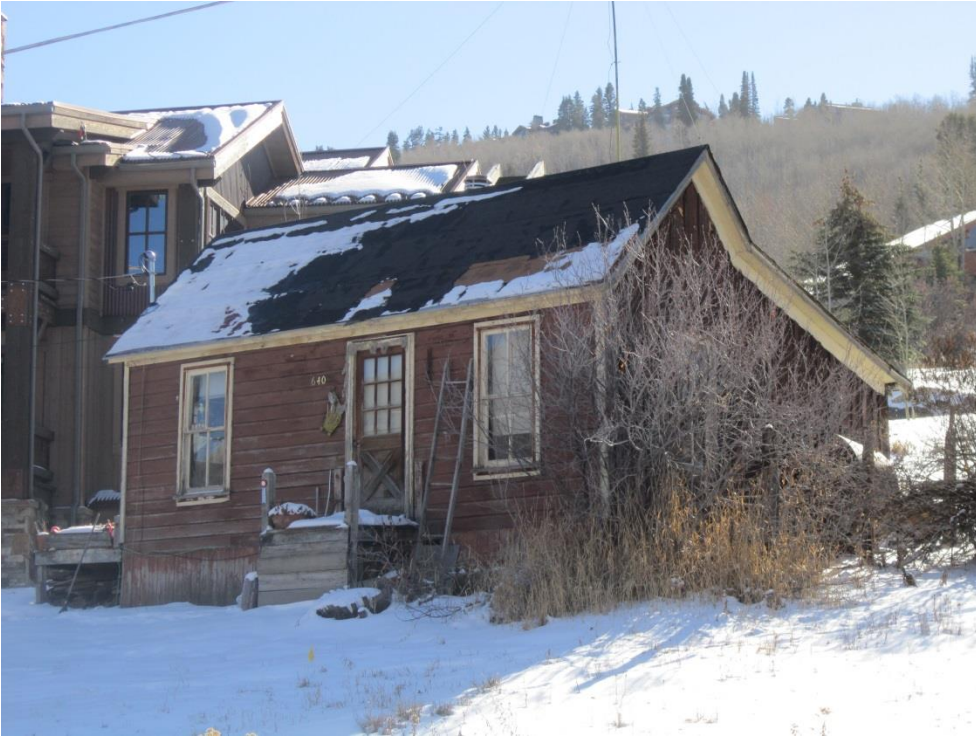
660 Rossie Hill Drive. Northwest oblique. November 2013.
