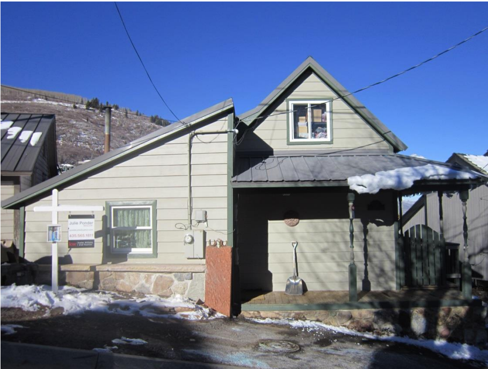
52 Prospect Street. West elevation. November 2013.
