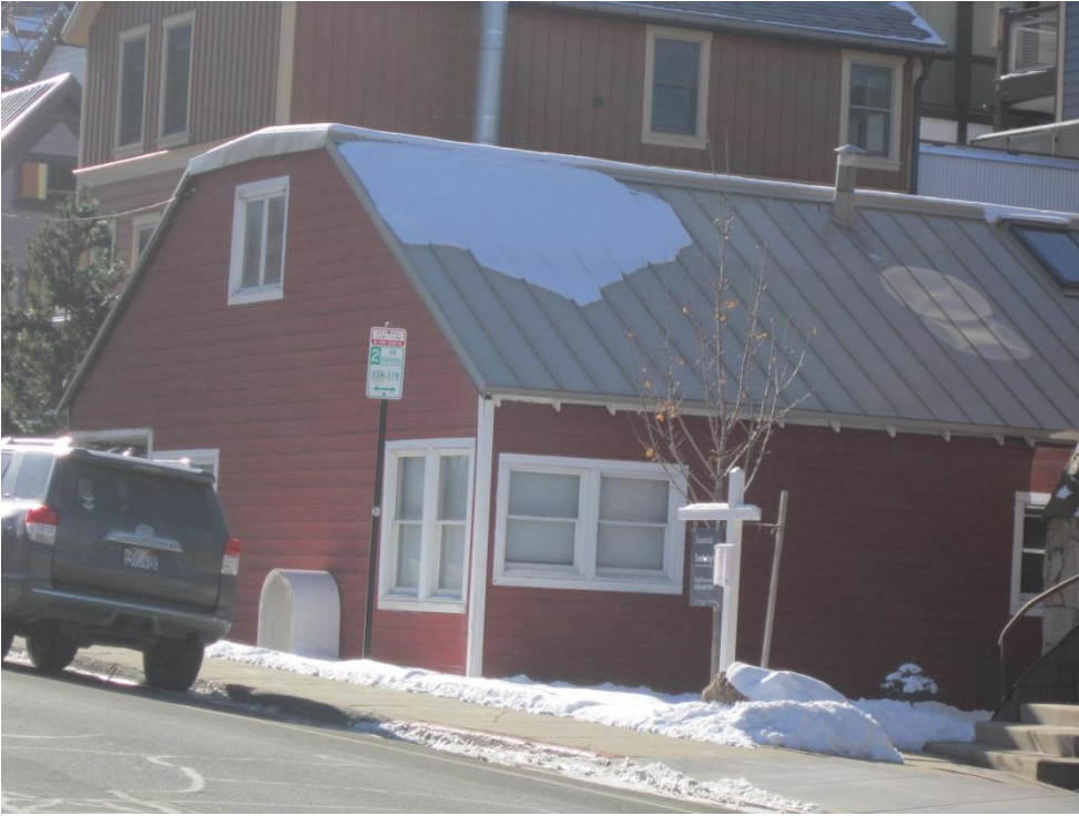
819 Park Avenue. Northeast oblique. November 2013.
