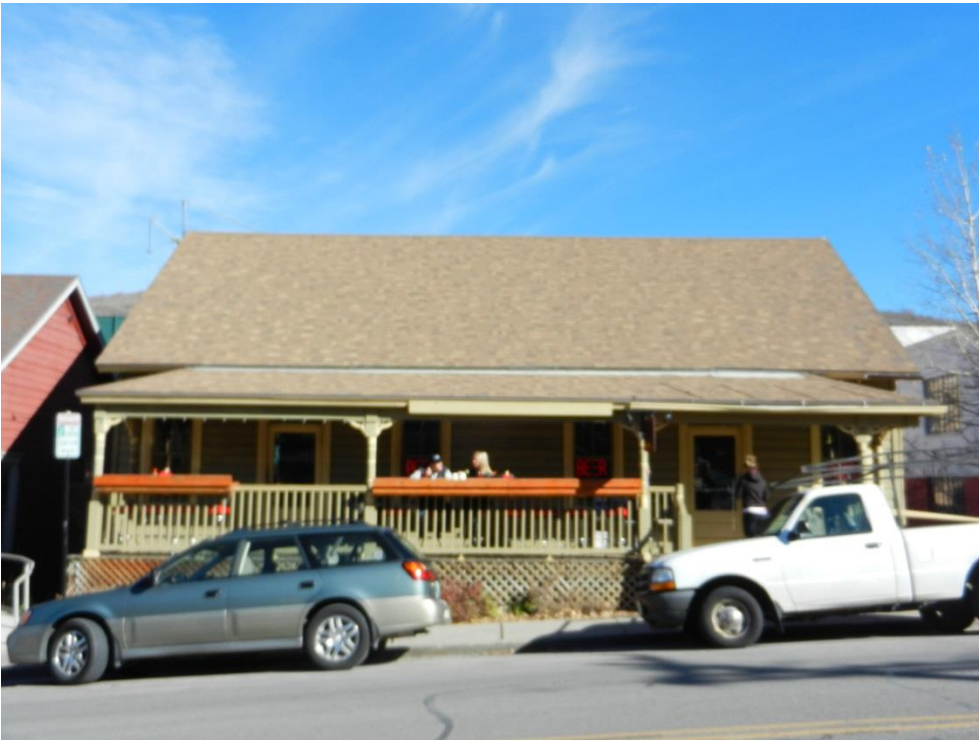
690 Park Avenue. West elevation. November 2013.
