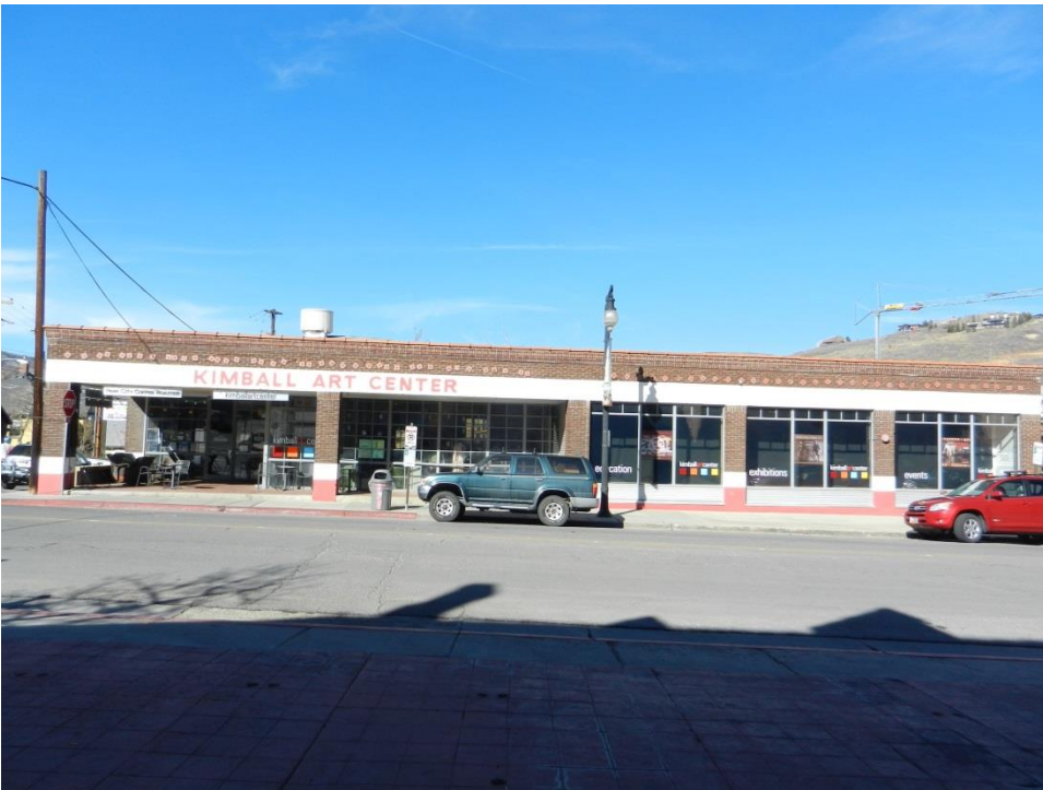
638 Park Avenue. South elevation. November 2013.
