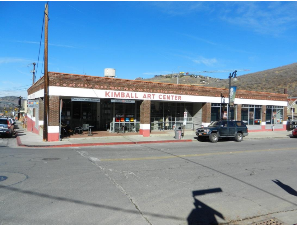
638 Park Avenue. Southwest oblique. November 2013.
