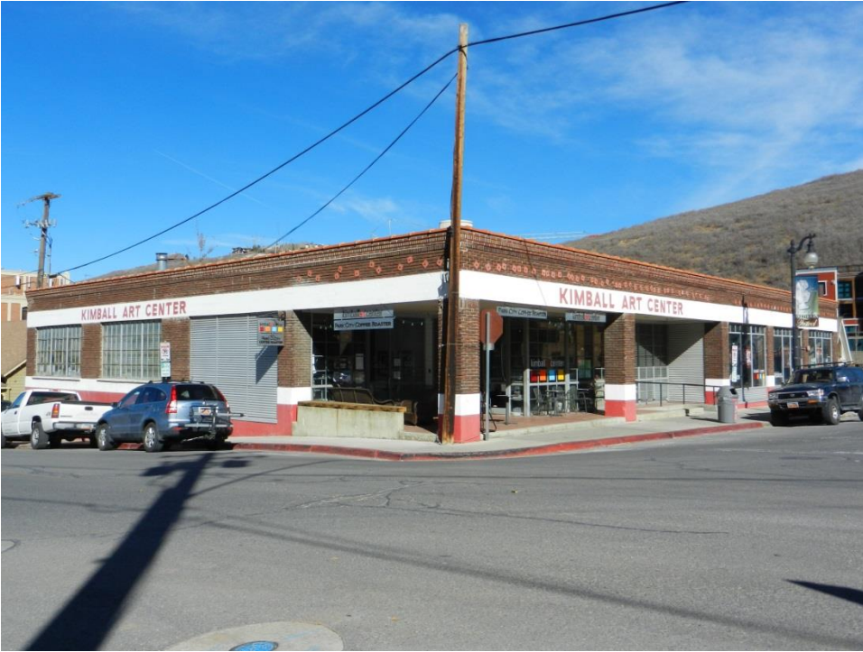
638 Park Avenue. Southwest oblique. November 2013.
