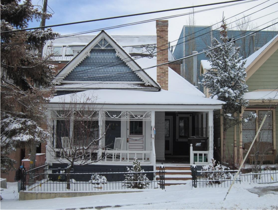
614 Park Avenue. West elevation. November 2013.
