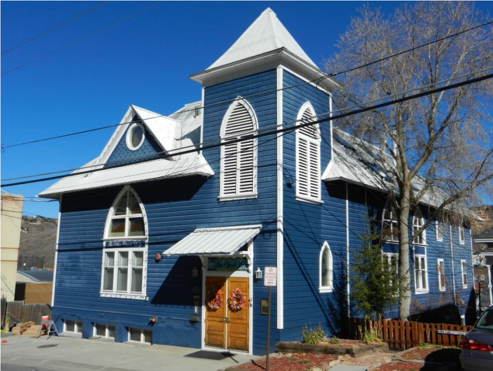
424 Park Avenue. Southwest oblique. November 2013.
