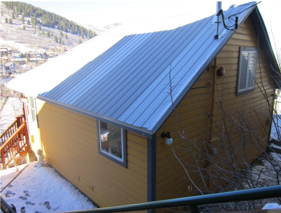
405 Ontario Avenue. Southeast oblique. November 2013.
