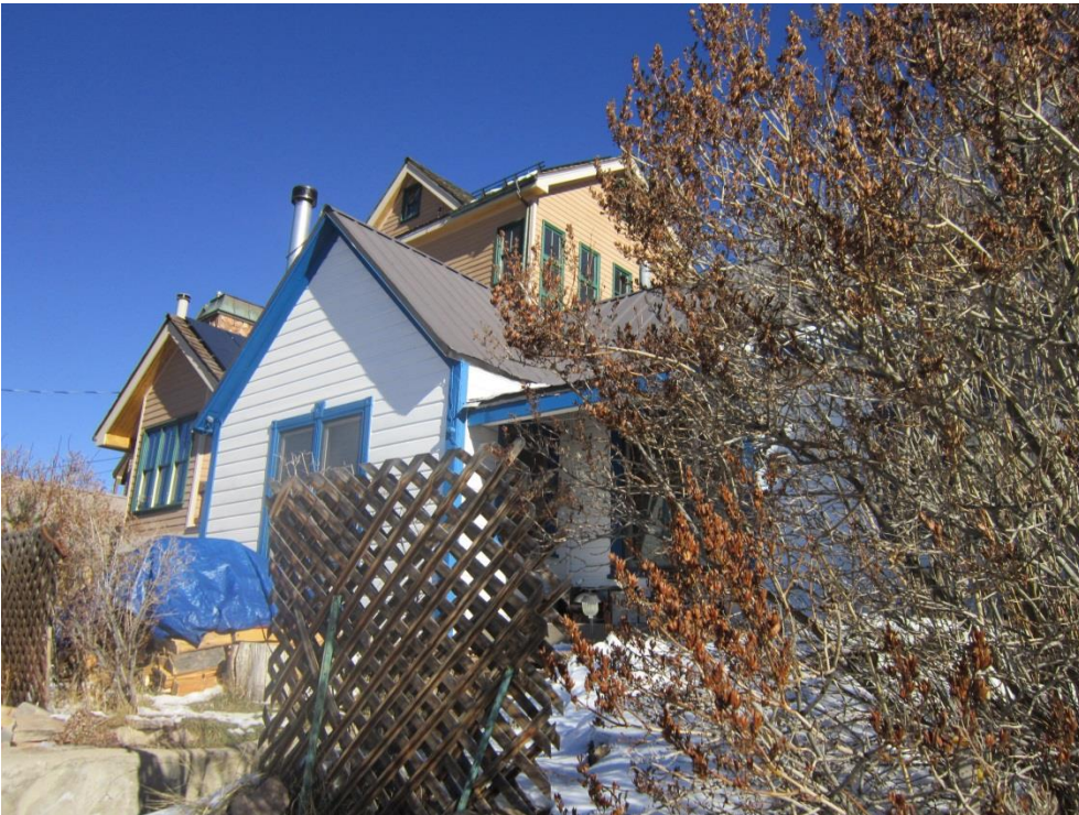
323 Ontario Avenue. Southwest oblique. November 2013.
