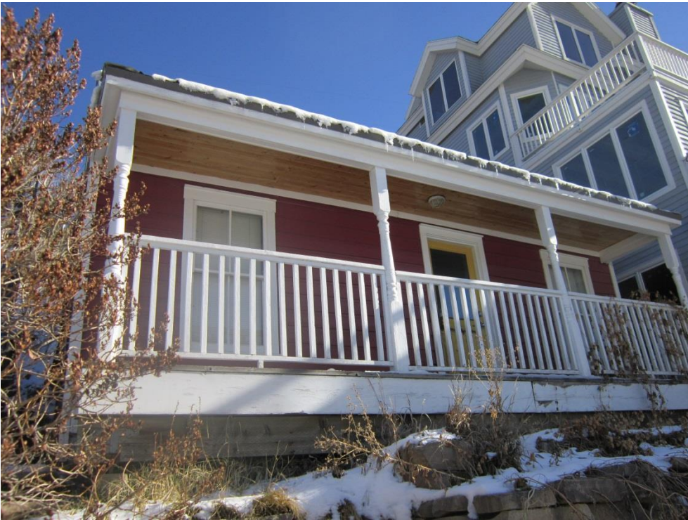
317 Ontario Avenue. West elevation. November 2013.
