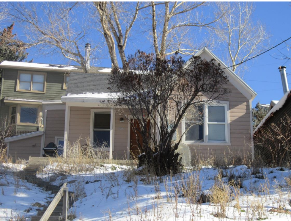
316 Ontario Avenue. West elevation. November 2013.
