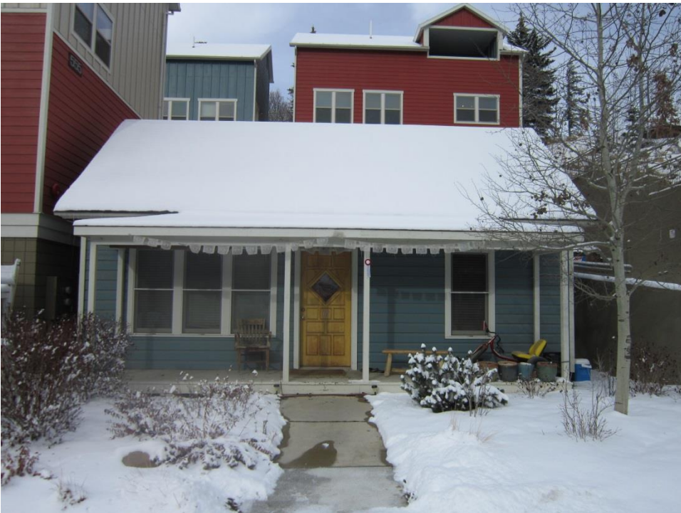
577 Deer Valley Drive. South elevation. November 2013.
