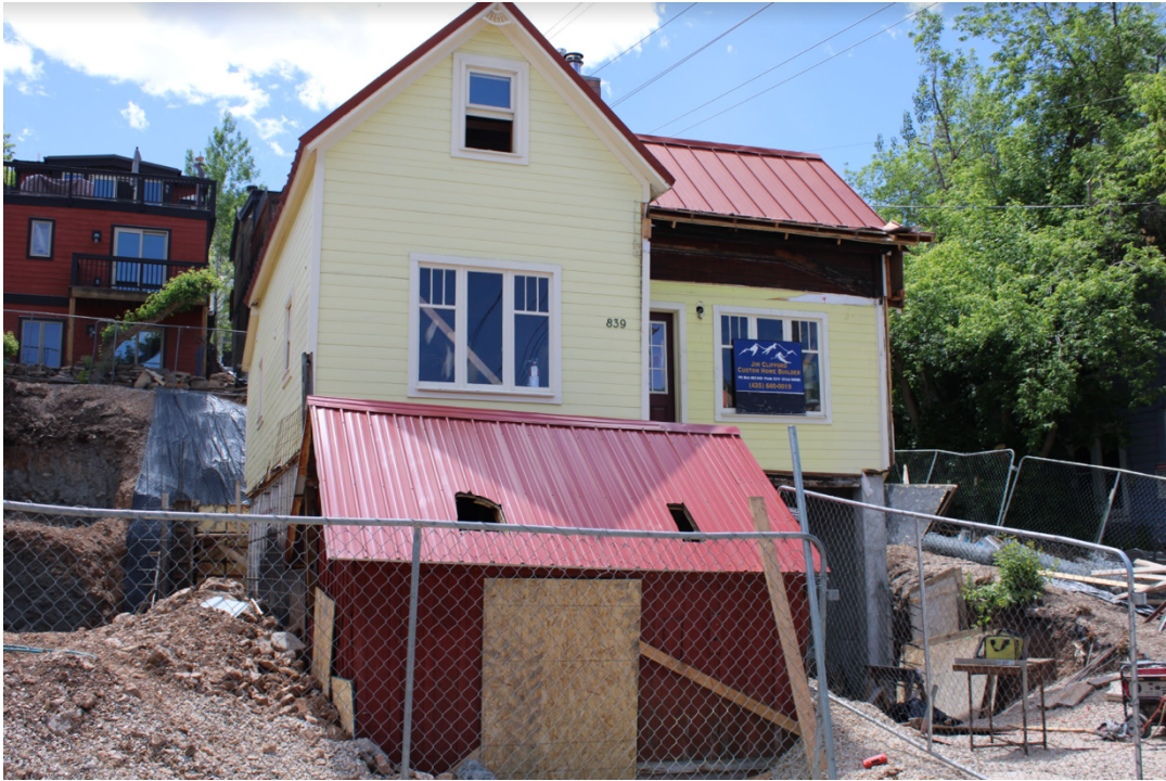
Photo 1: 839 Woodside Avenue. East elevation. 2020
