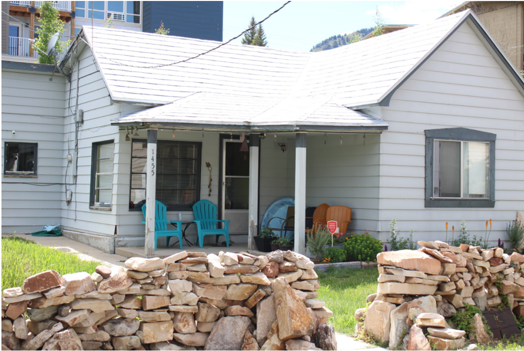
Photo 1: 1455 Woodside Avenue. Southeast oblique. 2020
