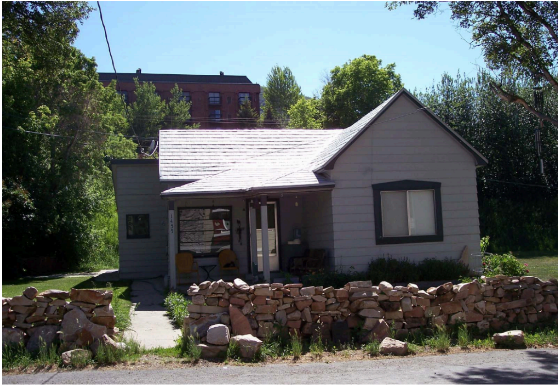
Photo 5: 1455 Woodside Avenue. East elevation. 2006
