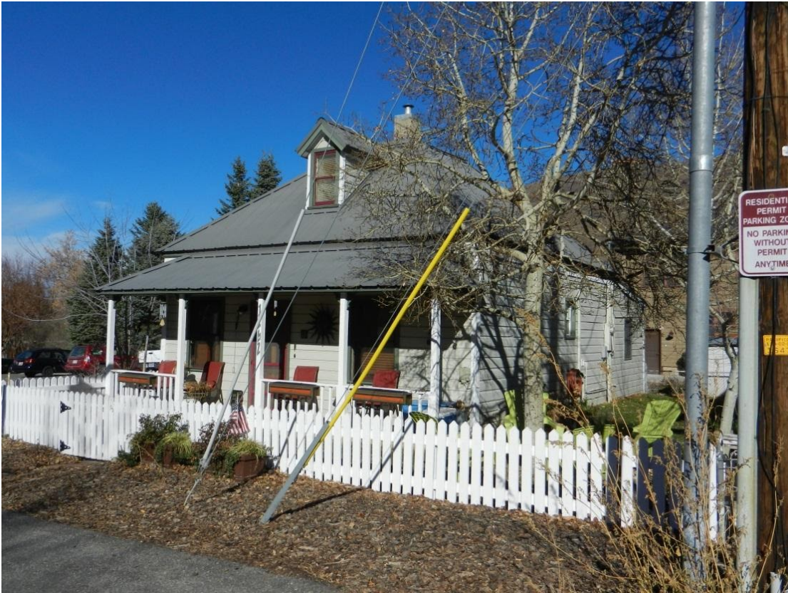
Photo 2: 1162 Woodside Avenue. Southwest oblique. November 2013
