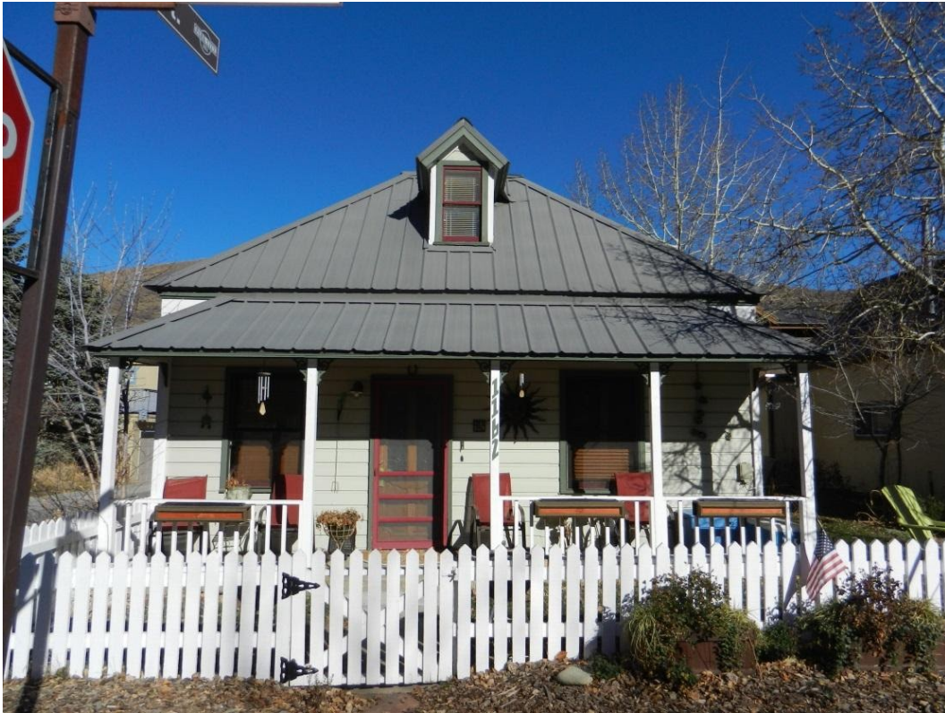
Photo 3: 1162 Woodside Avenue. West elevation. November 2013
