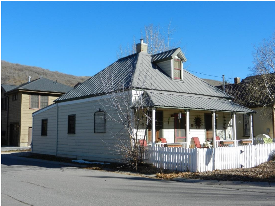
Photo 4: 1162 Woodside Avenue. Northwest oblique. November 2013
