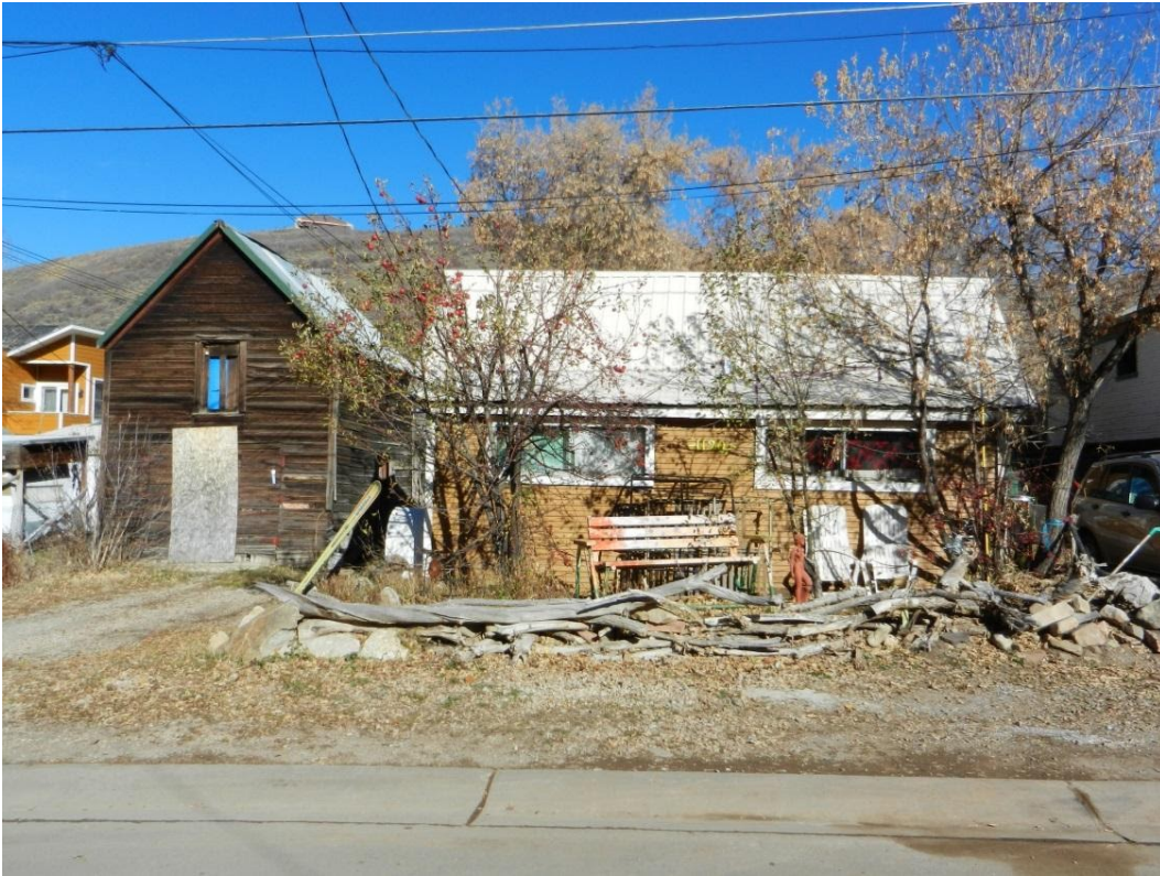
Photo 3: 1120 Woodside Avenue. West elevation. November 2013
