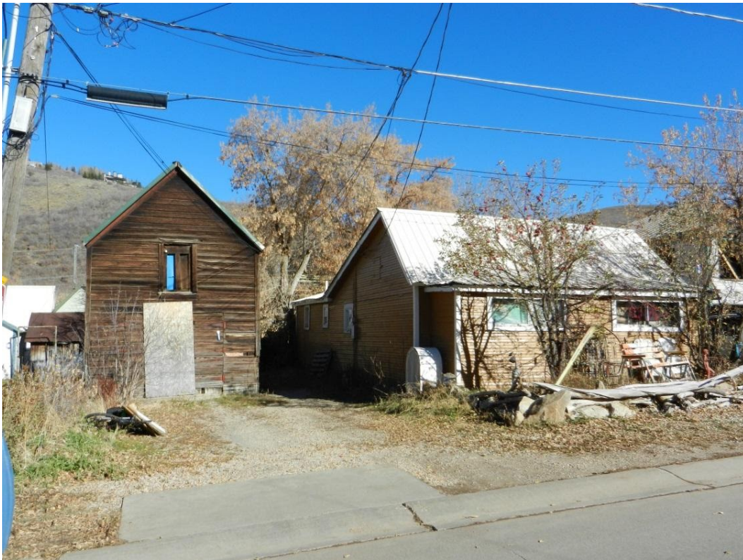
Photo 4: 1120 Woodside Avenue. Northwest oblique. November 2013
