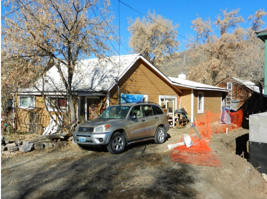
Photo 2: 1120 Woodside Avenue. Southwest oblique. November 2013
