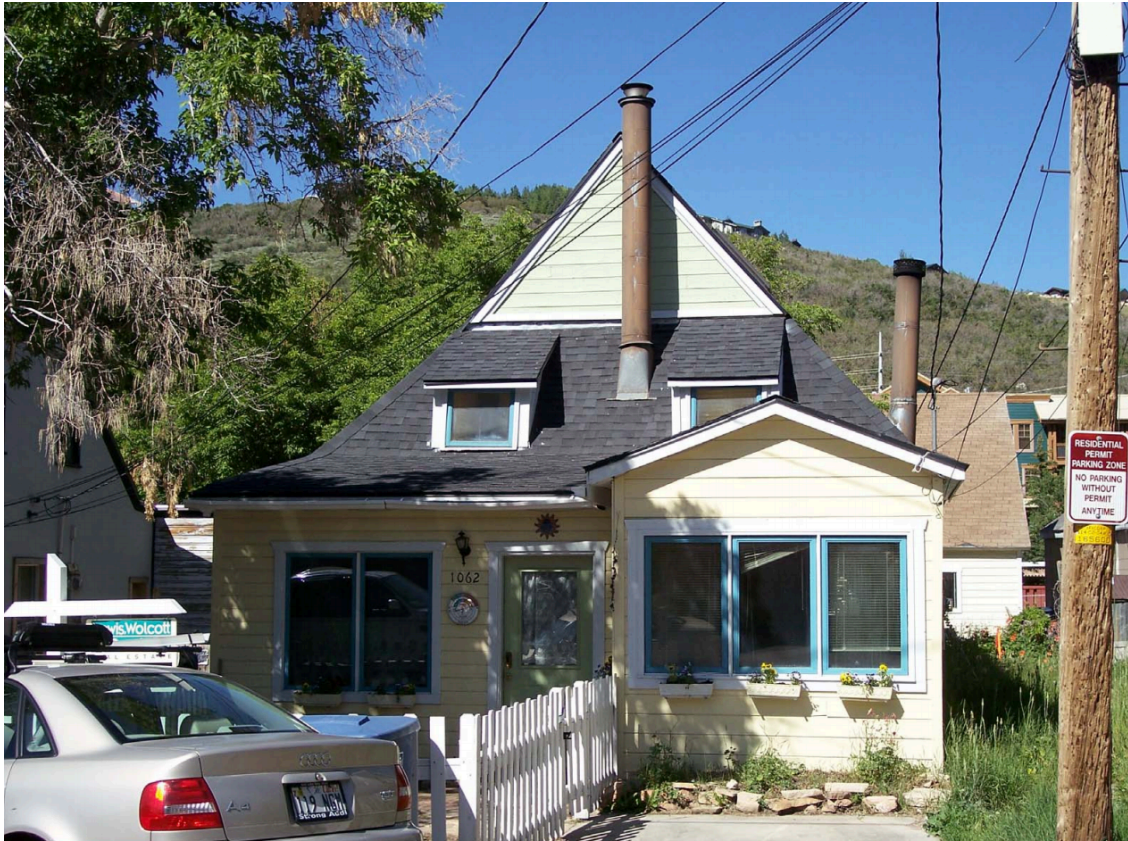
Photo 5: 1062 Woodside Avenue. West elevation. 2006
