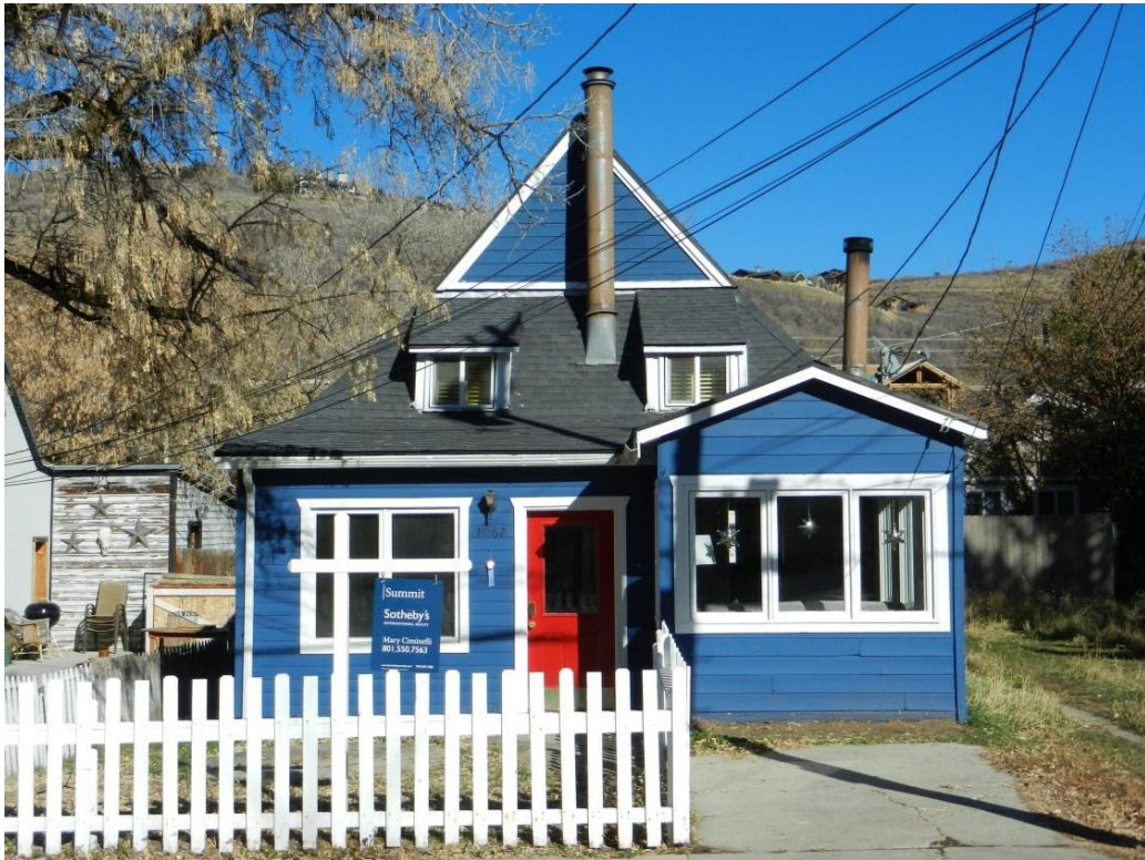
Photo 3: 1062 Woodside Avenue. West elevation. November 2013
