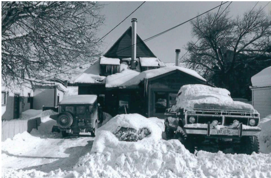
Photo 6: 1062 Woodside Avenue in 1981 (Historic Architectural Survey, 1982)
