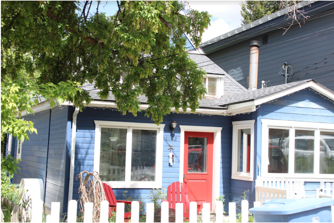
Photo 1: 1062 Woodside Avenue. Northwest oblique 2020
