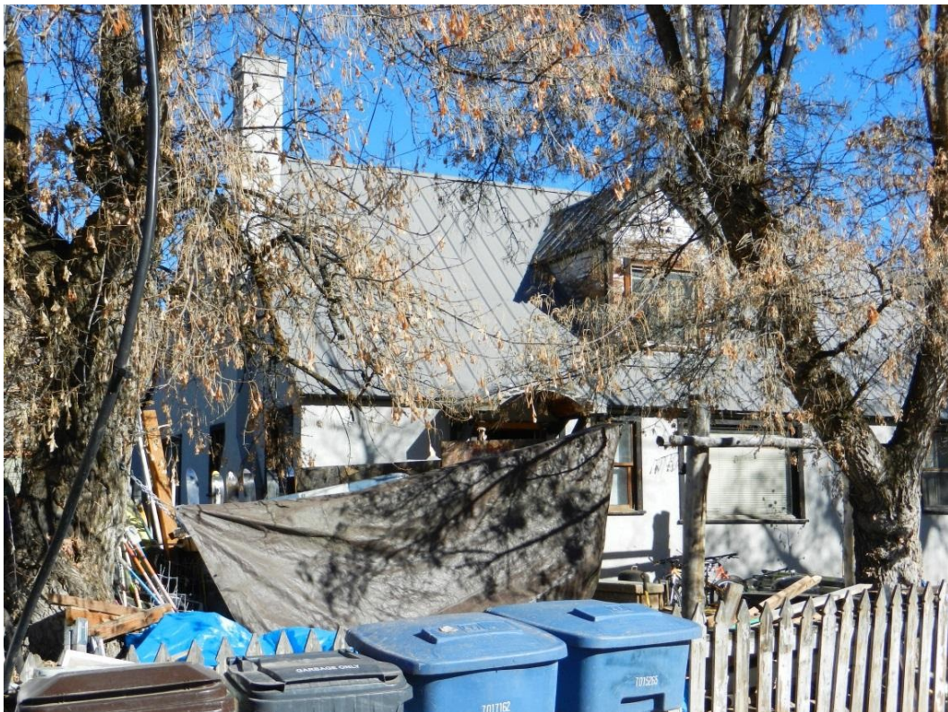
Photo 4: 1060 Woodside Avenue. Northwest oblique. November 2013
