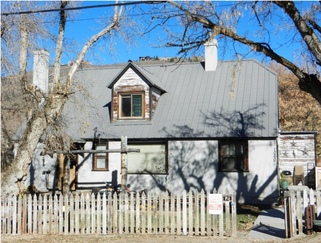
Photo 3: 1060 Woodside Avenue. West elevation. November 2013
