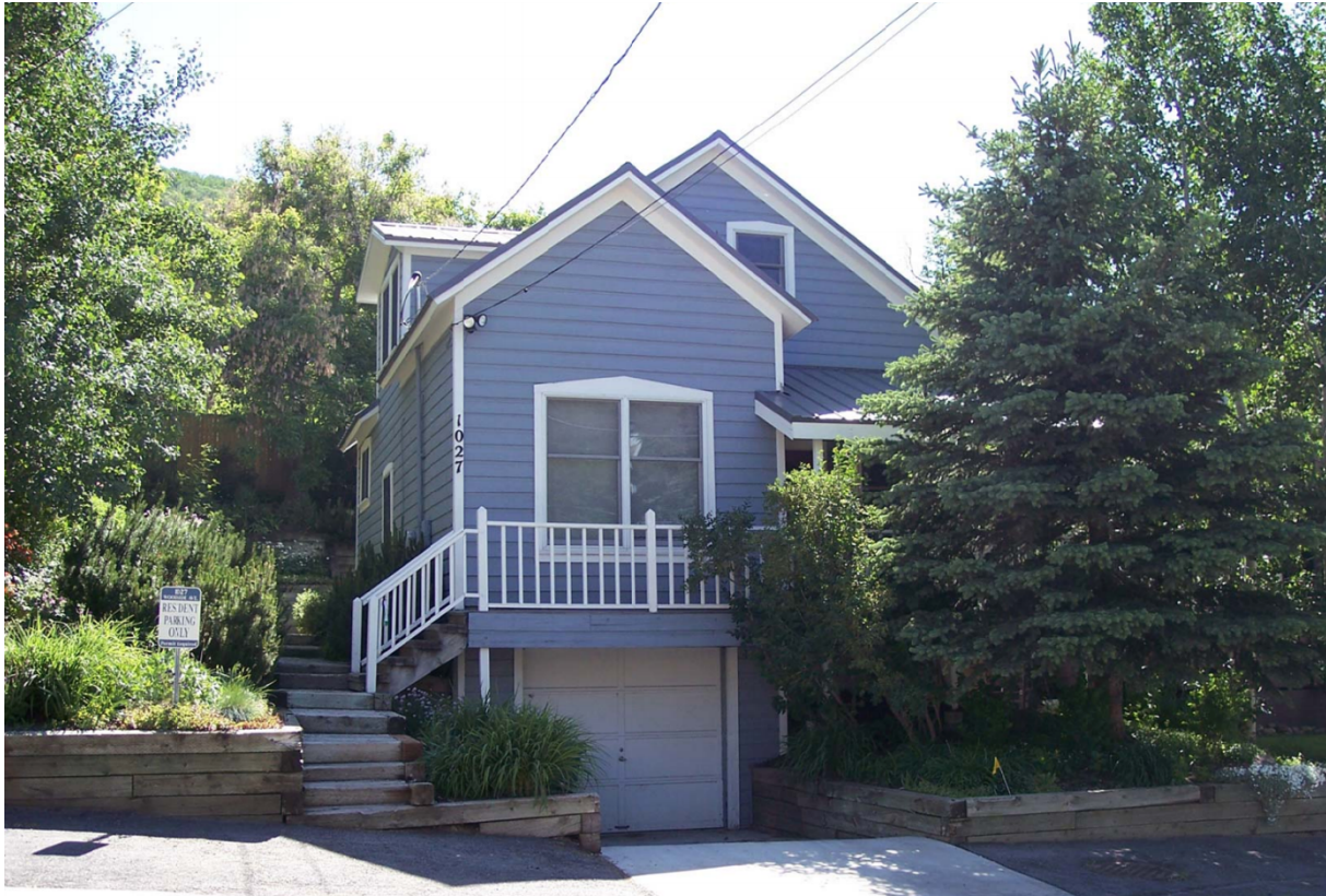
Photo 5: 1027 Woodside Avenue. Southeast oblique. 2006
