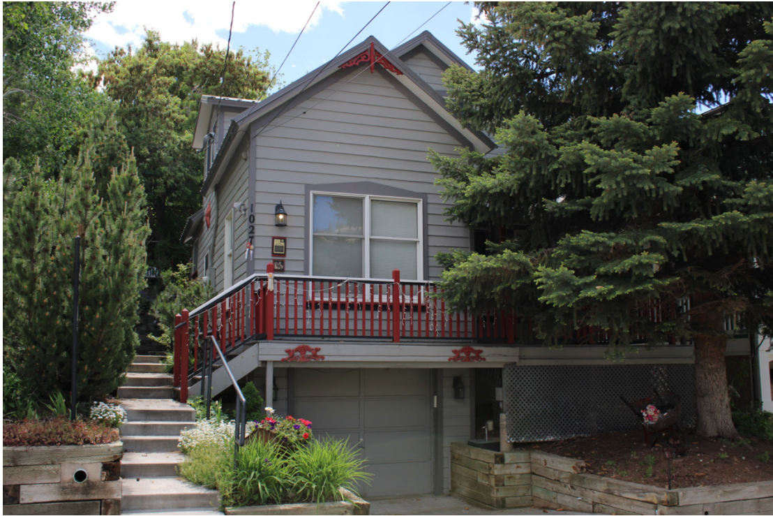
Photo 1: 1027 Woodside Avenue. East elevation. 2020
