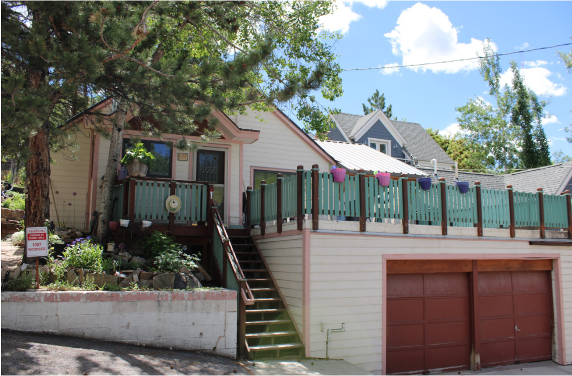
Photo 1: 1007 Woodside Avenue. East elevation. 2020
