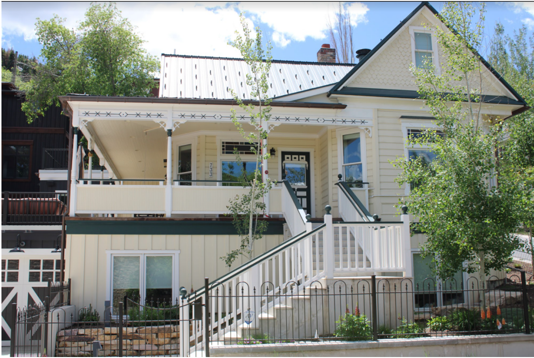
Photo 1: 733 Woodside Avenue. East elevation. 2020
