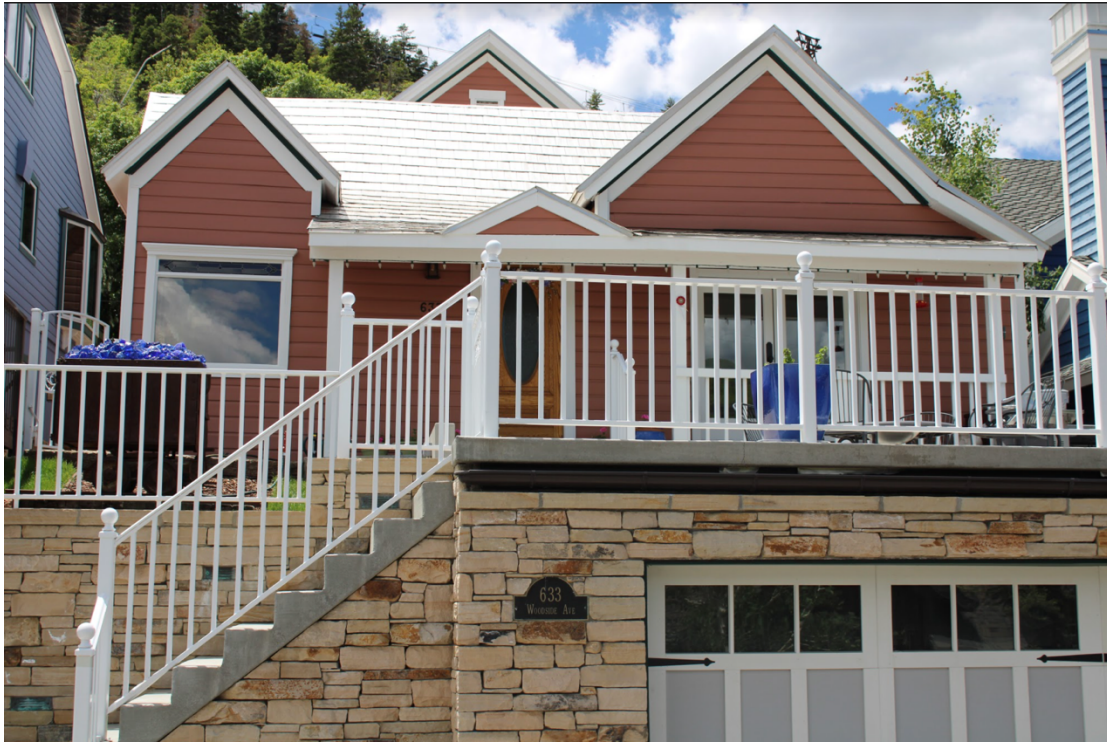
Photo 1: 633 Woodside Avenue. East elevation. 2020
