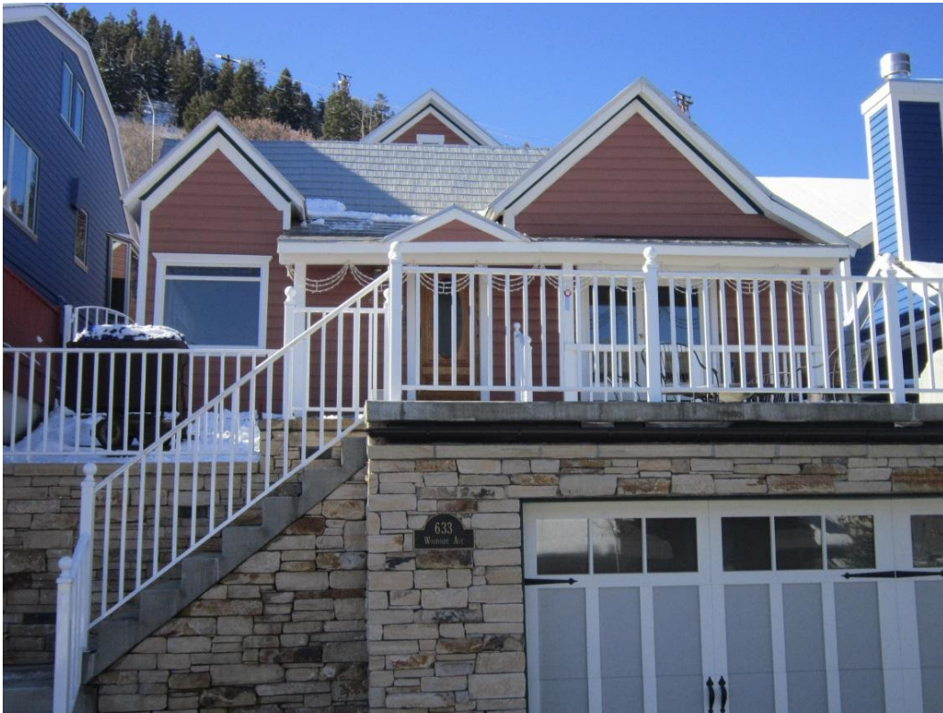
Photo 3: 633 Woodside Avenue. East elevation. November 2013
