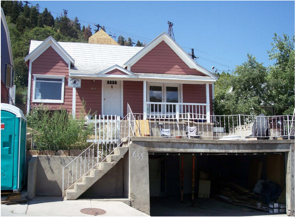
Photo 5: 633 Woodside Avenue. East elevation. 2006
