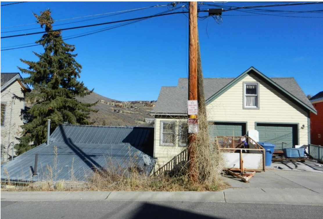
Photo 2: 424 Woodside Avenue. West elevation. November 2013
