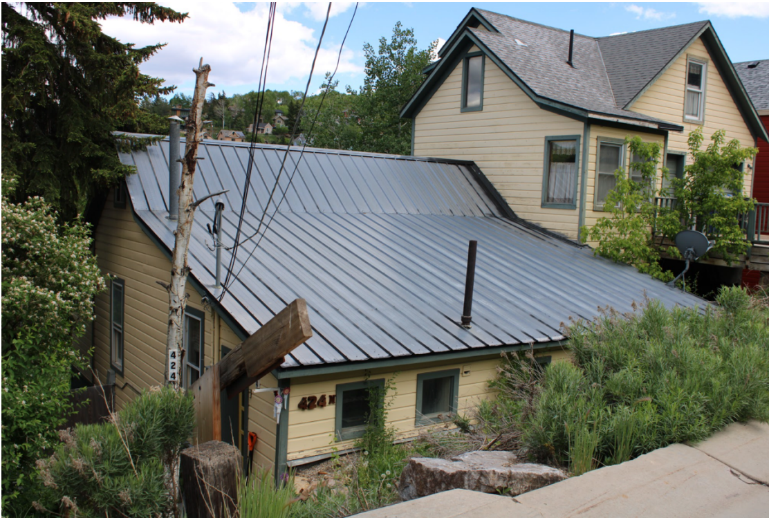
Photo 1: 424 Woodside Avenue. Northwest oblique. 2020
