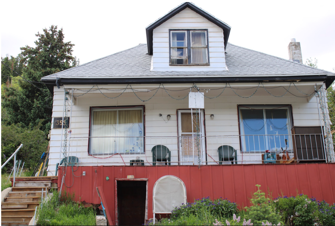
Photo 1: 359 Woodside Avenue. East elevation. 2020
