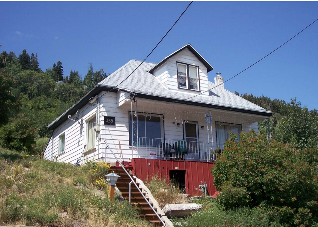
Photo 4: 359 Woodside Avenue. Southeast oblique.2006
