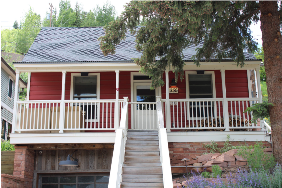
Photo 1: 335 Woodside Avenue. East elevation. 2020
