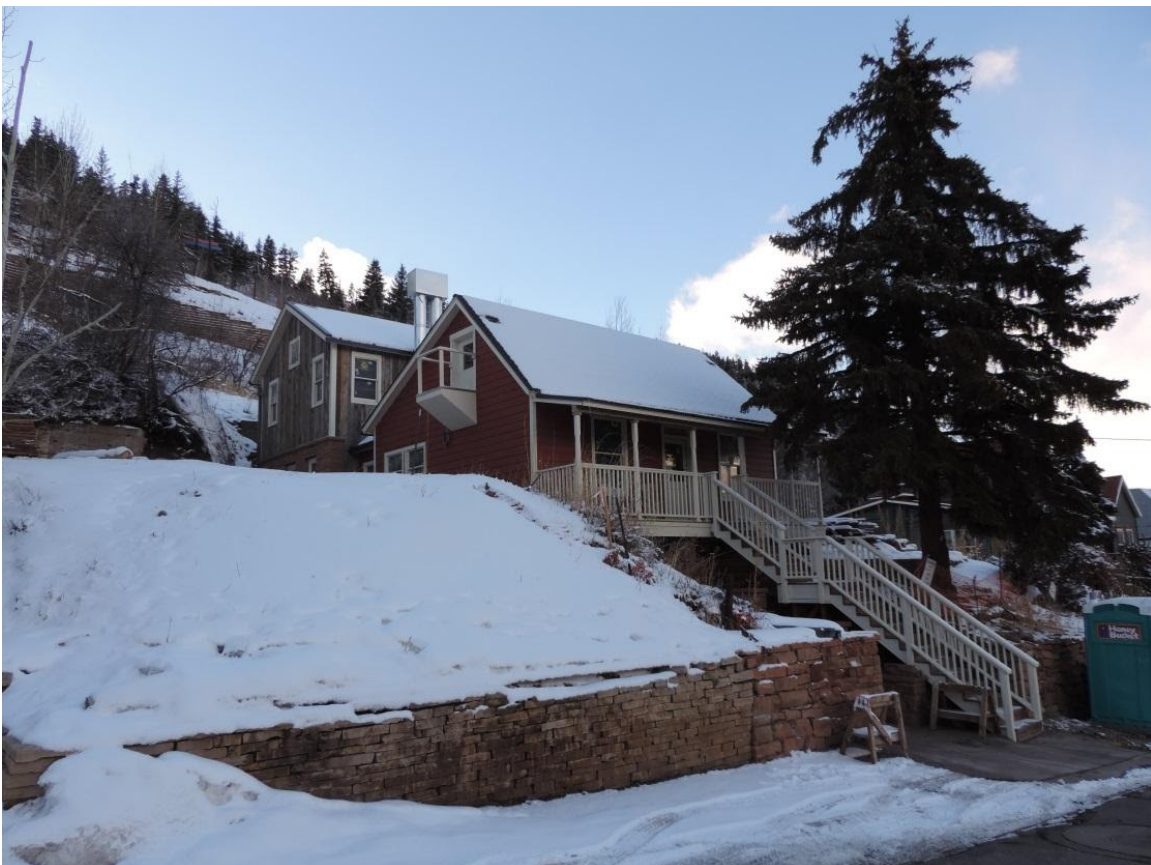
Photo 2: 335 Woodside Avenue. Southeast oblique. December 2015
