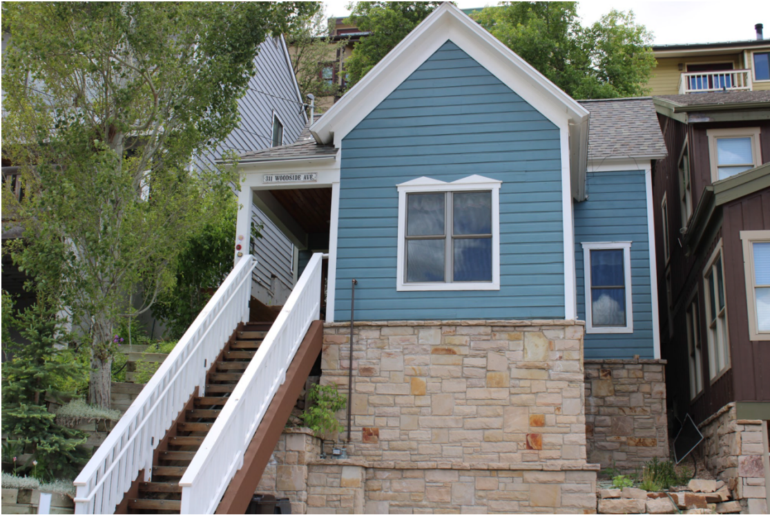
Photo 1: 311 Woodside Avenue. East elevation. 2020
