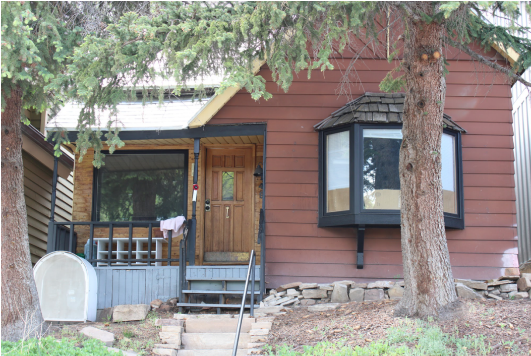
Photo 1: 149 Woodside Avenue. East elevation. 2020
