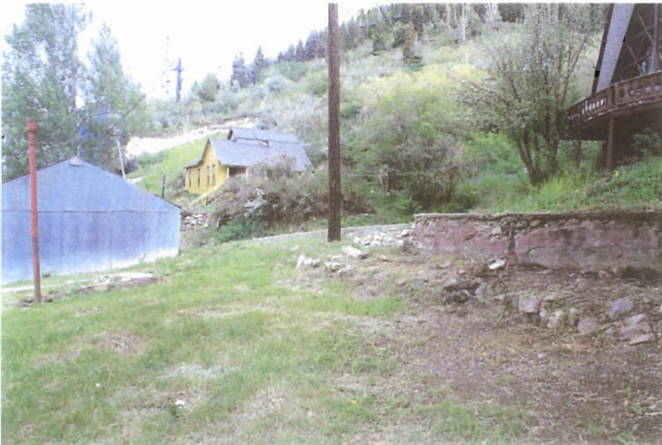
Retaining wall at top west side of property
