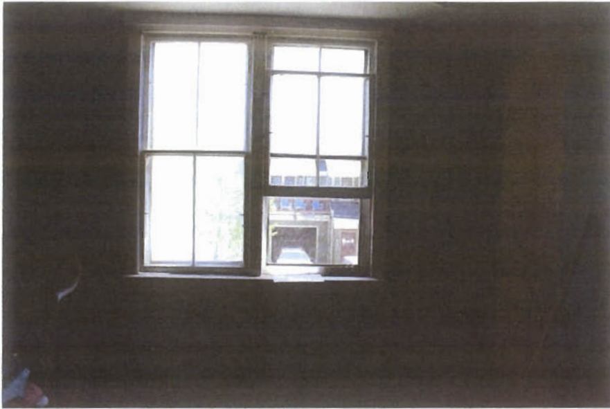
East window pair from interior. 1X4 at head and jambs. 1X sill with 1X4 apron. 3/4" muntin.
