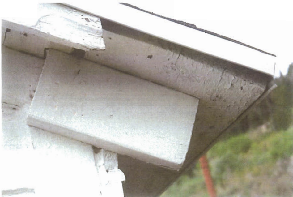
Overhang at northwest rear elevation- Note metal drip edge
