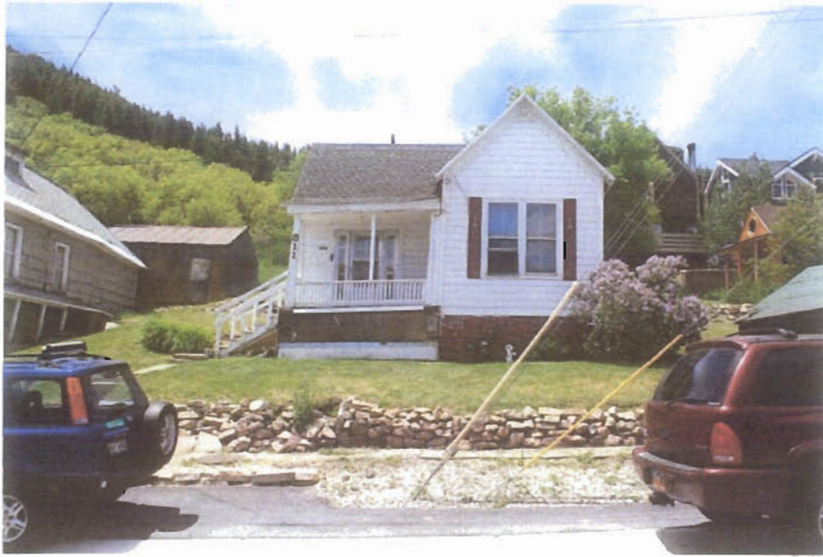
Retaining wall at front-east elevation
