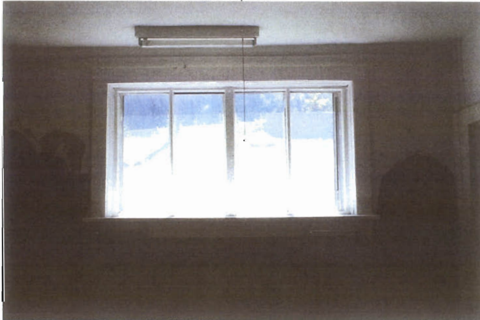
Interior kitchen window 1X4 trim, \frac{3}{4} " sill and 1X4 apron
