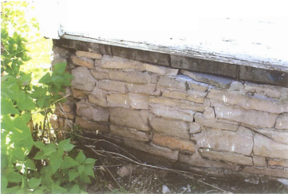
Unreinforced stone foundation- joist bearing
