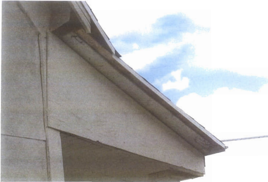
Porch roof intersection with south gable
