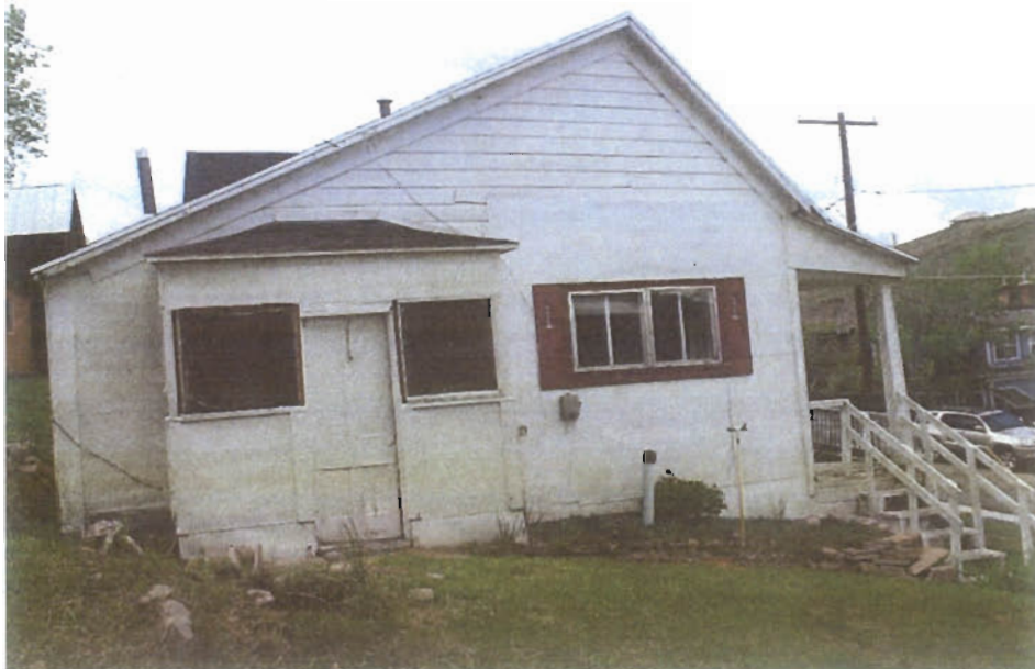
Back entry door 30" wX 6'-4 1/2" h stile and rail panels larger on top-simplified from interior door
