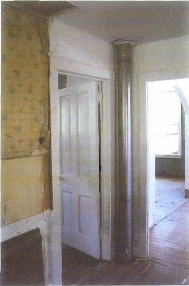
Typical door and trim. Arched opening seen beyond.
