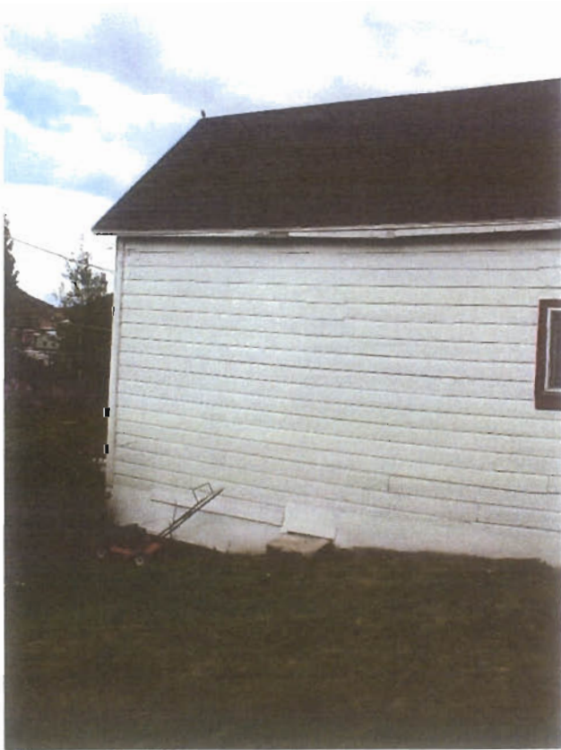
Change in 1X4 trim at ? chimney
