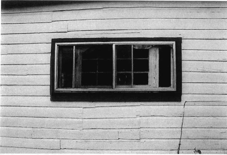
Evidence of original window
