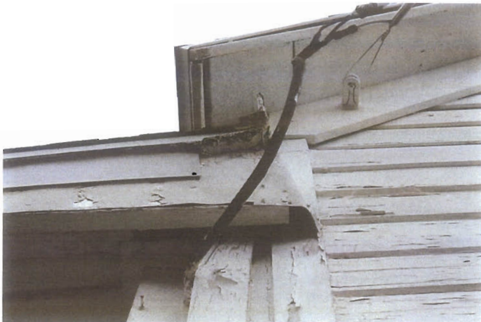
Intersection porch roof and gable roof east elevation
