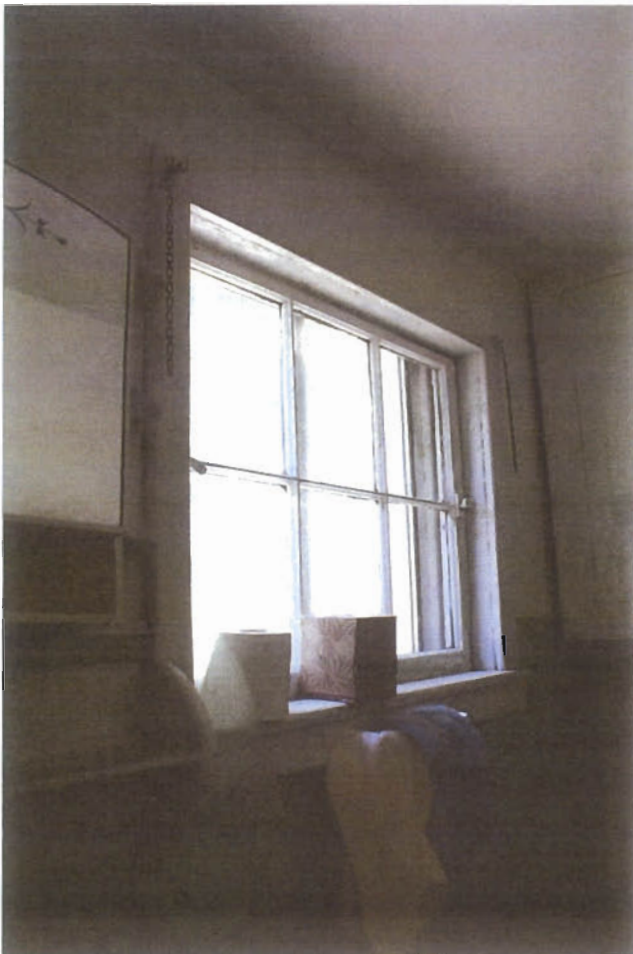
West bathroom window interior 1X4 trim with apron
