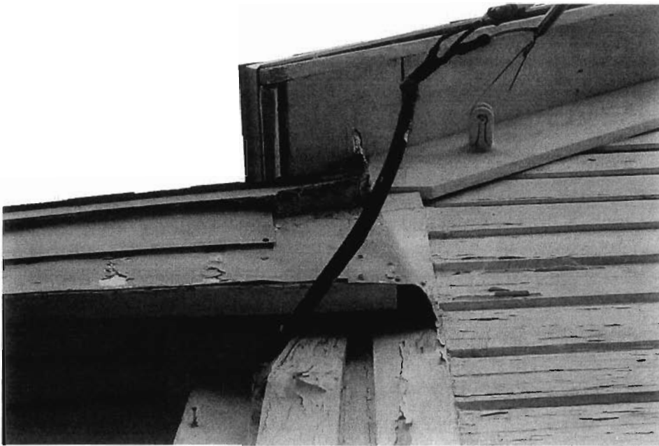
Double wall between gable and porch
