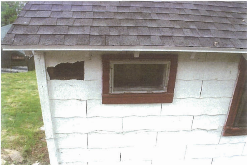
West window added later than 1911.
