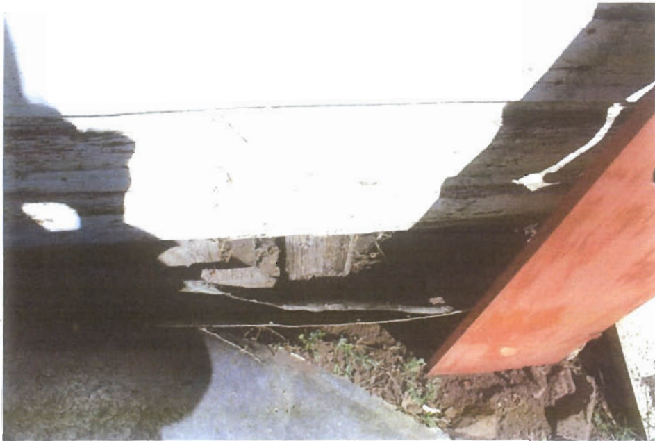
Wood on earth pony wall foundation-joist bearing
