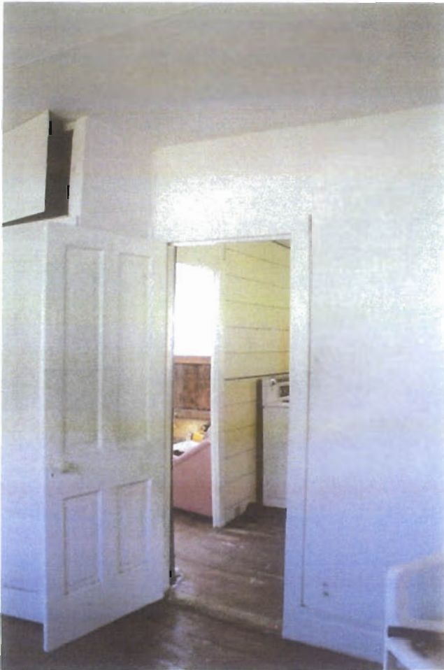
Interior door are all 4 paneled doors with a larger upper panel width and height vary
