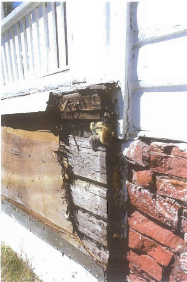
Unreinforced, stone foundation
