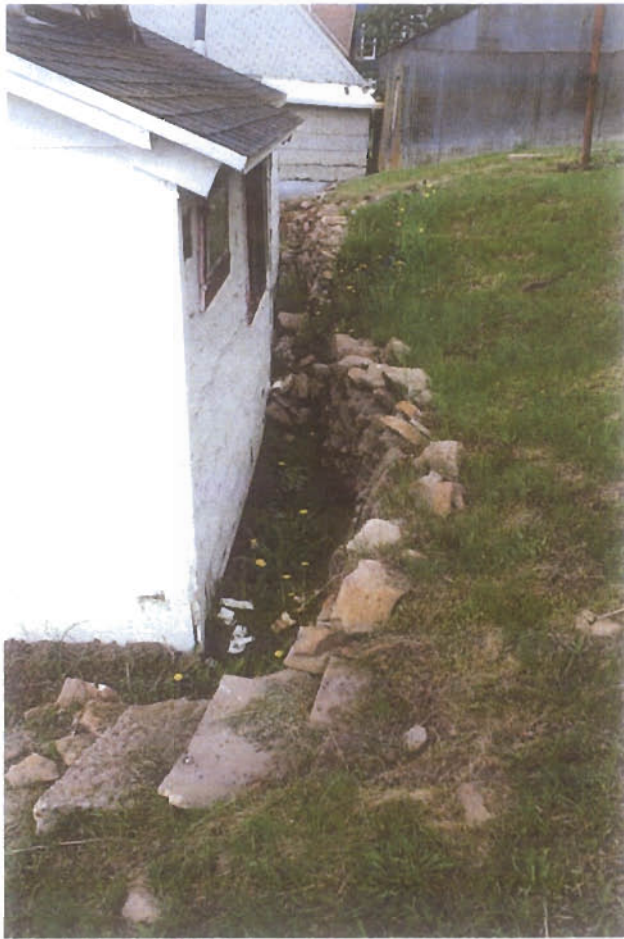
Retaining wall behind house north to south
