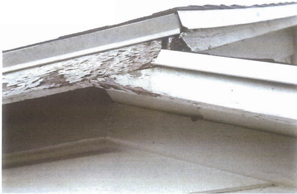
Intersection gable roof to shed roof on north elevation
