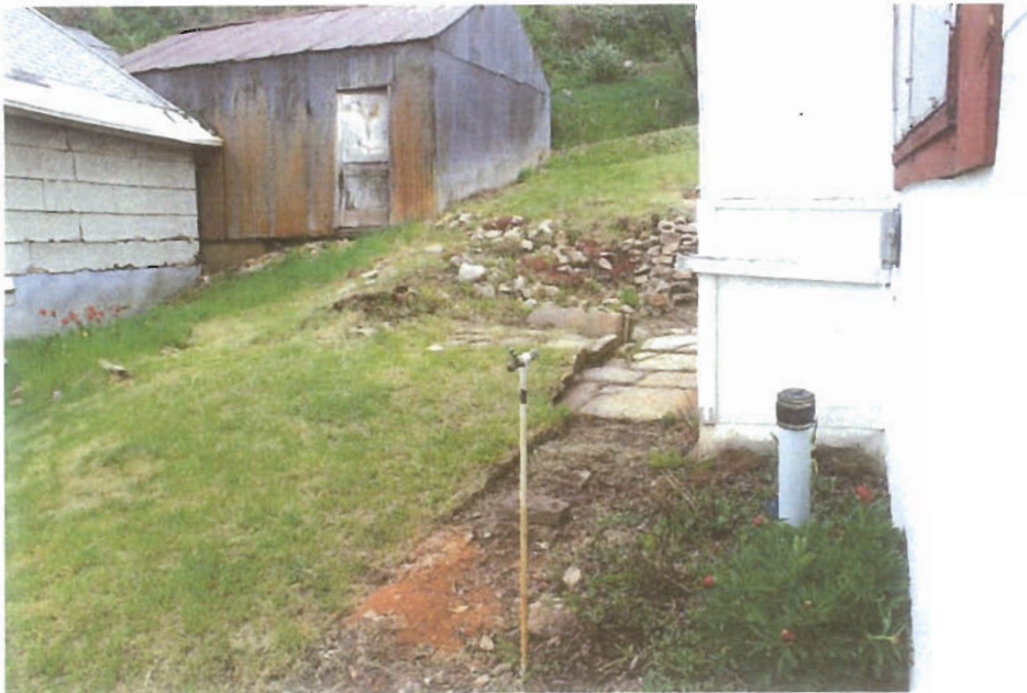
Water main turnoff
