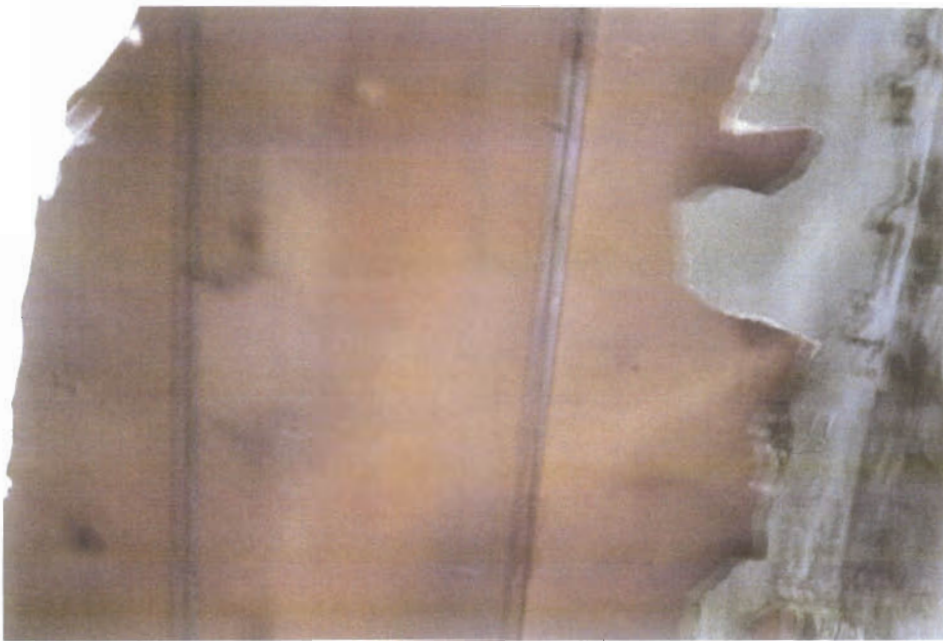
1X12 planks at ceiling
