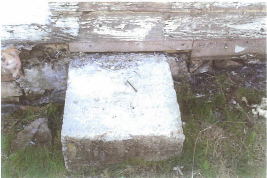
Concrete pad/foundation North Elevation
