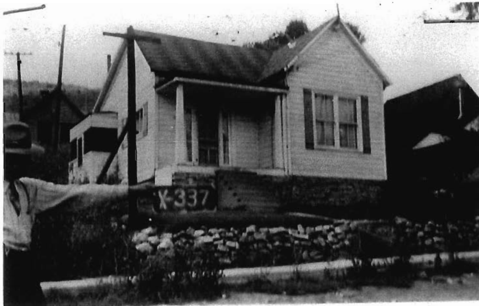
1937 Historic Tax Photo-front east retaining wall
