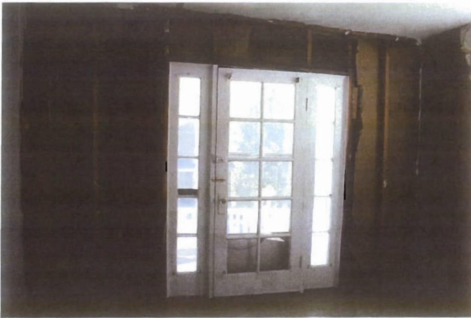
East facing front door and sidelights
