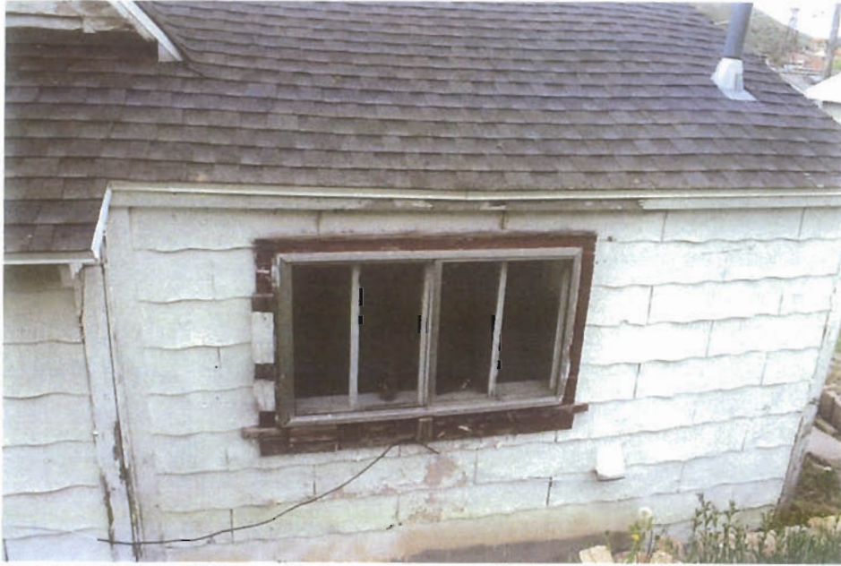
West elevation kitchen window casement (2) 1" muntin with single divided pattern 3'-10"wX2'-6"h 4'-1" off the ground 1X4 trim with extended 1X sill and apron
