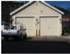
Across from Transit Center Trash and Cardboard Recycling Compactors
