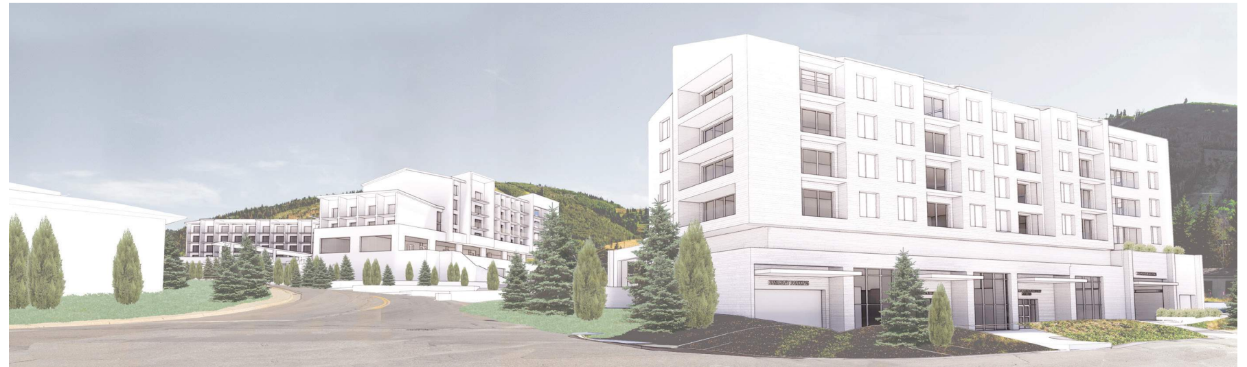
View from northeast corner of Parcel E (Parcel C at left)
