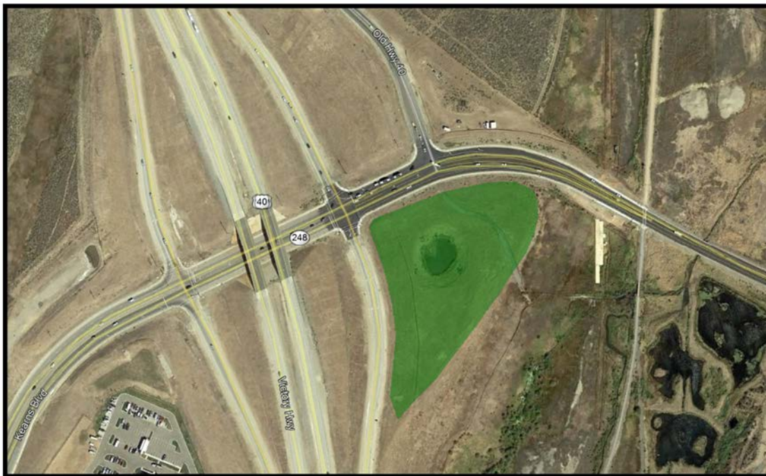
Figure 4 - UDOT Detention Basin Site- (Source: Google Earth)
