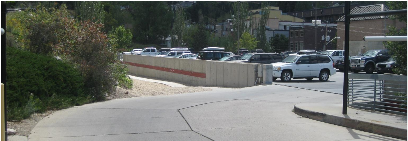
Figure 14: Tight Curve to China Bridge Garage Upper Level
