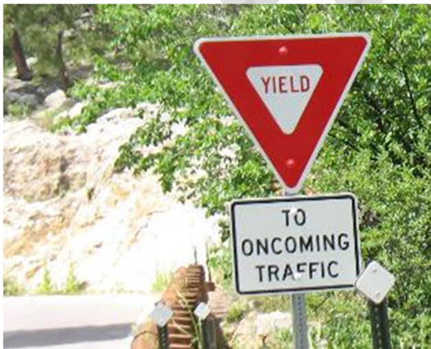
Figure 6: Example of Yield Sign and Supplementary Plaque – Wind Cave National Park, SD
