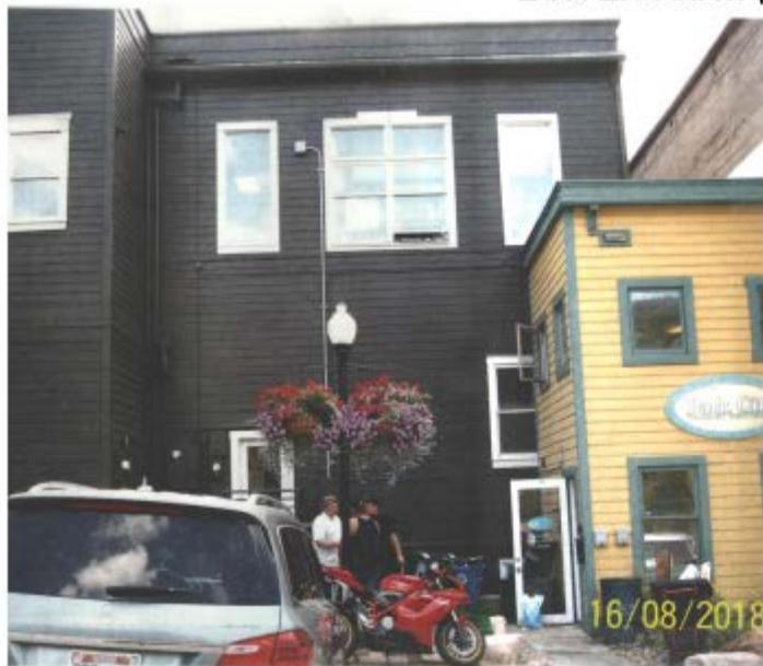
Existing Swede Alley Façade
